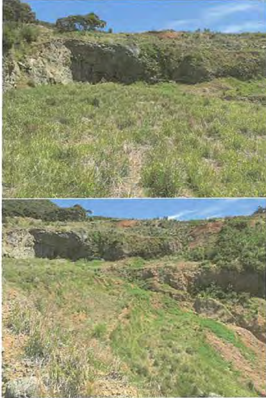
Stage 3 Rehabilitation site
