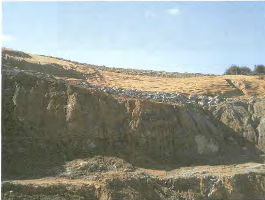
Photograph (ii) Environmental cloth laid down
