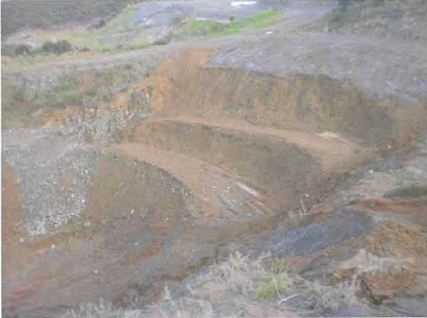
Photograph (VI). Stage 3 overburden stockpile site benched and “slash” laid out on top level. As the overburden disposal site is filled to the finished levels slash will be applied to promote growth.
