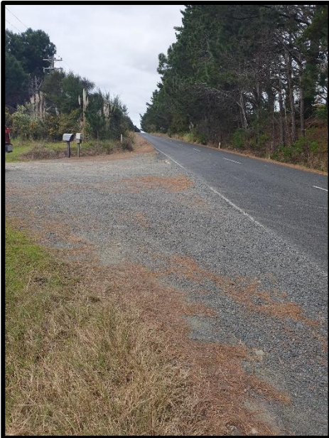
Figure 17: Existing crossing from the access lot to Hihi Road.
