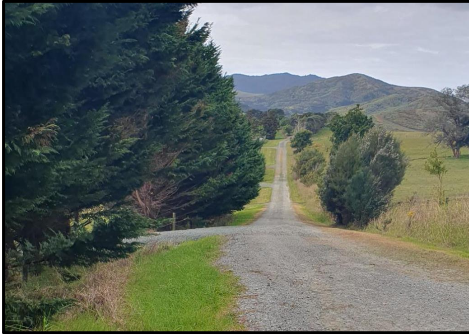
Figure 15: Existing carriageway within the access lot, showing the location of crossing places along the access lot.
