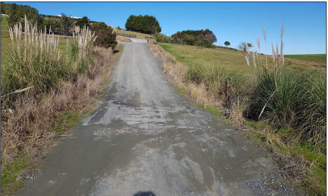
Figure 5 access looking south
