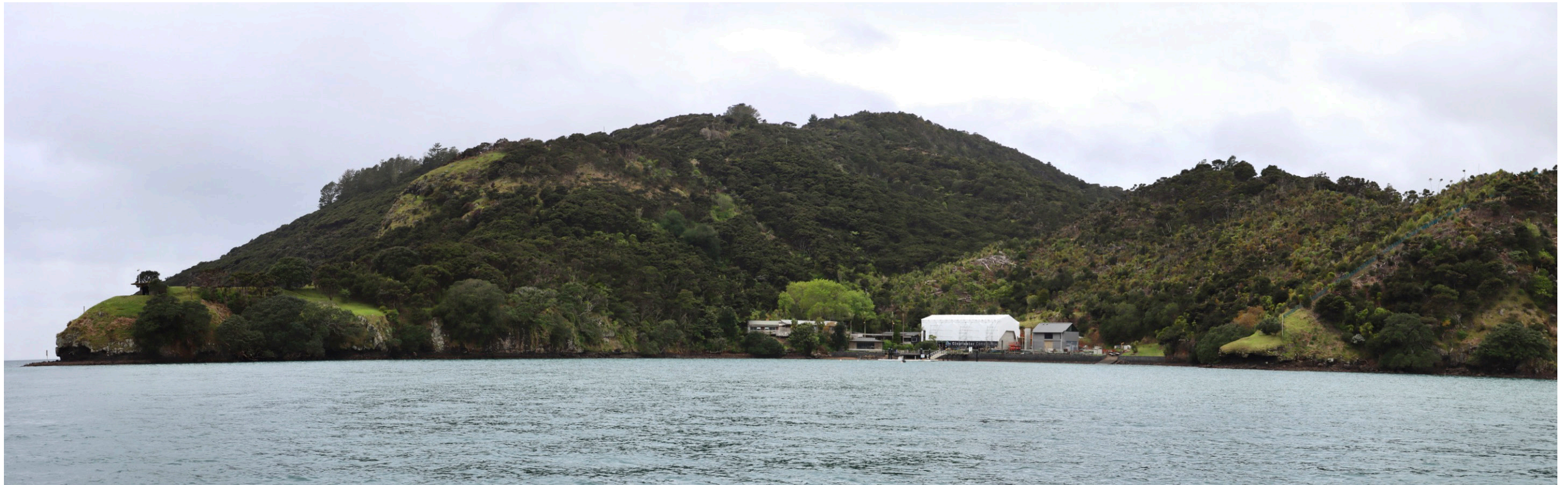
Viewpoint 5 - Looking towards Kingfish Lodge from the main boating channel towards the south
