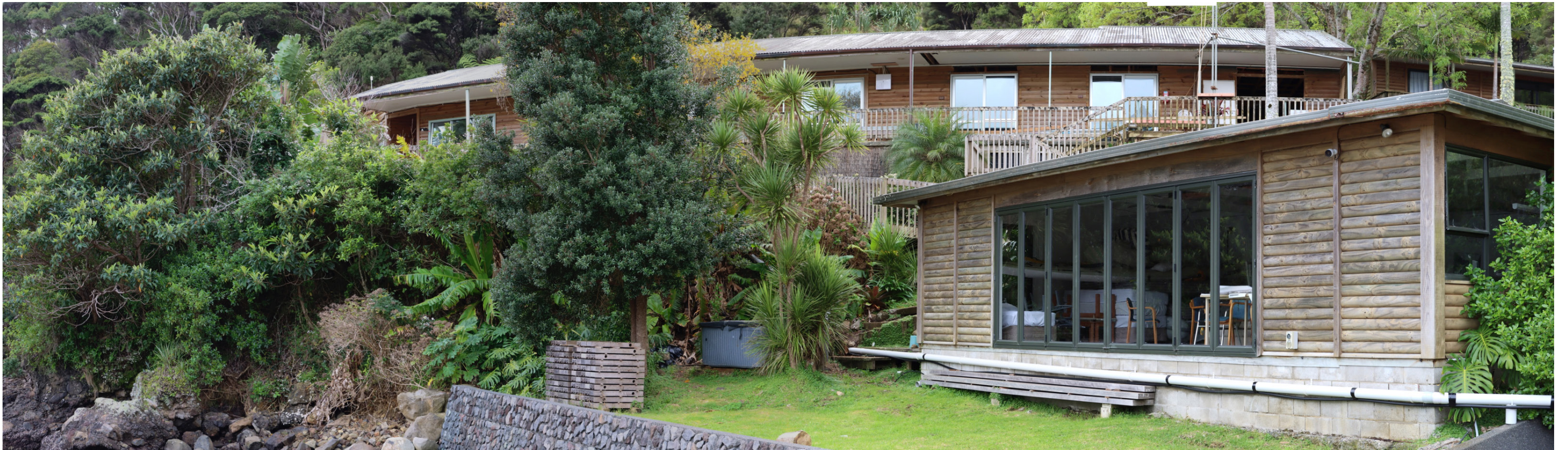
Photo 1 - View of the existing accomodation wing and conference room from the existing deck
