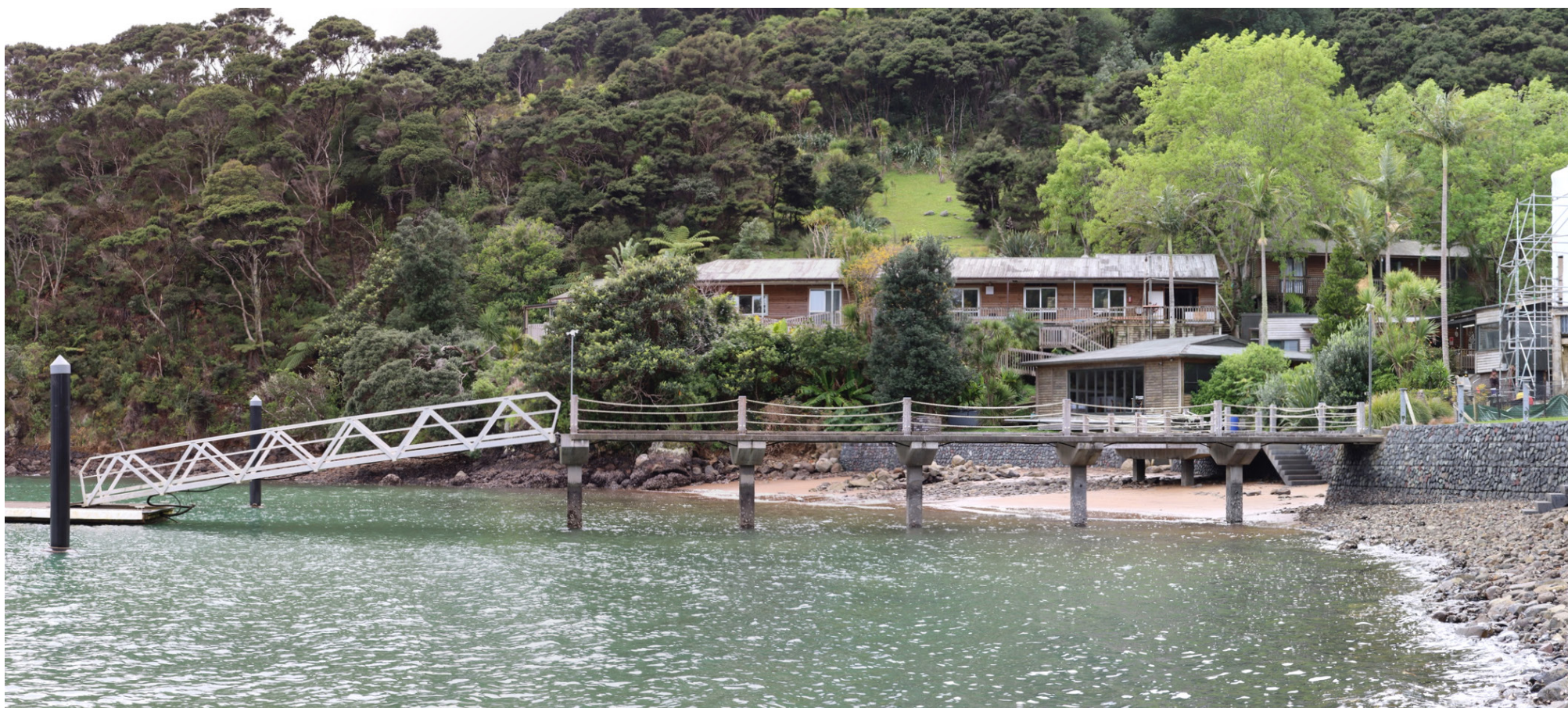
Photo 6 - View from the beach by the boat ramp at the southern end of the bay looking at the jetty, accomodation wing, conference room, deck, cottage, bar and restaurant area and the new Lodge under construction.
