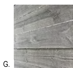
G. CONCRETE SHUTTER
