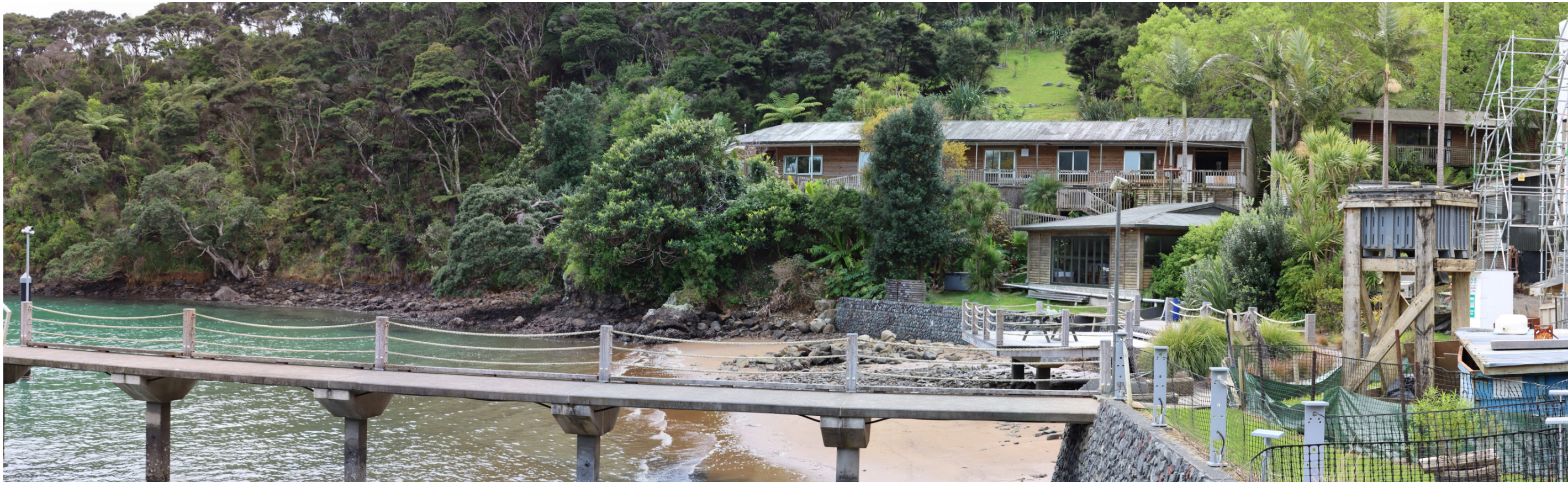
Photo 5 - View from the marginal strip of the jetty, accomodation wing, conference room, deck, bar and restaurant area and the new Lodge under construction.
