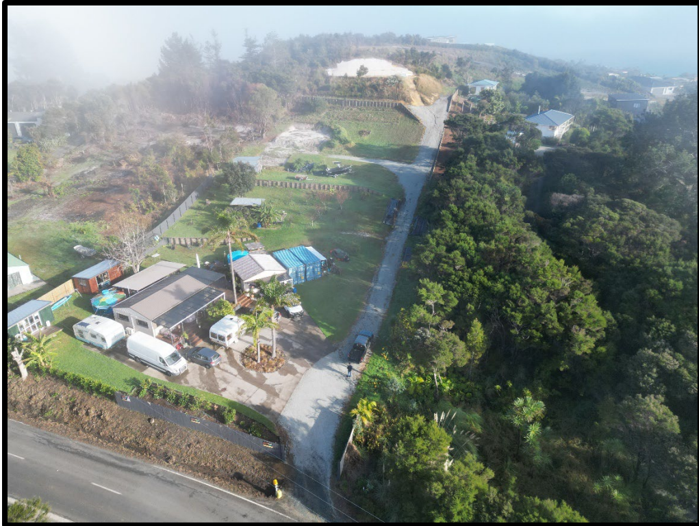
Figure 3: View of existing buildings and building platform
