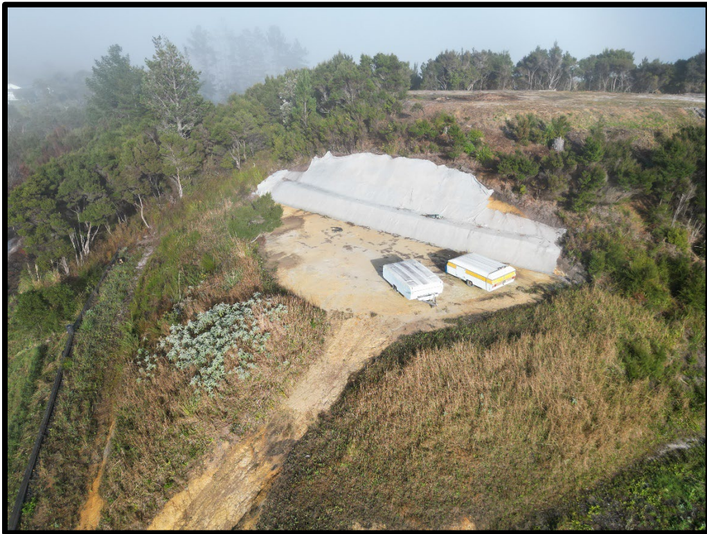
Figure 4: View of building platform
