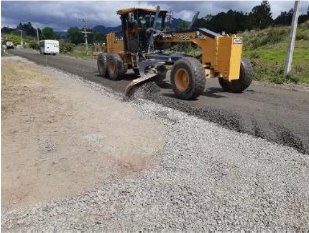
Omanaia Rd – Trimming of stabilised pavement
