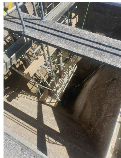
Kawakawa Clarifier Cleaning
