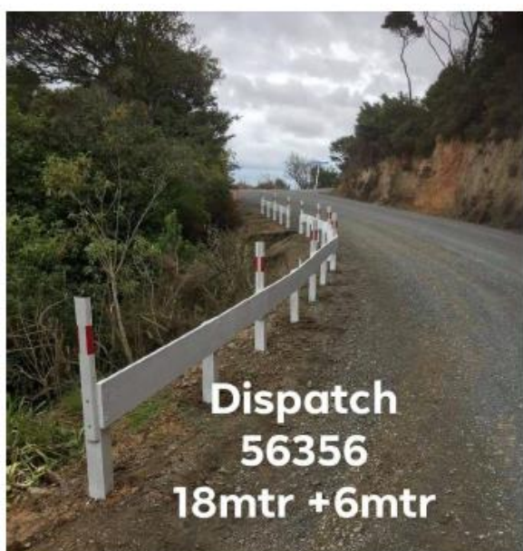
Haruru Falls Rd – Sight Rail Installation
