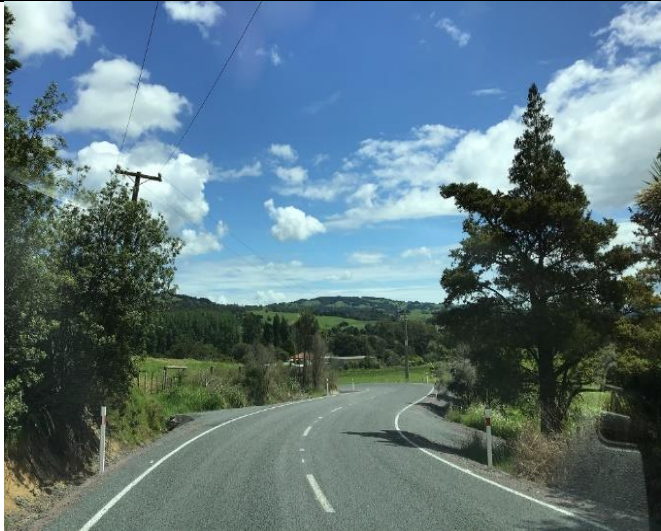
Puketi Seal Extension – Completed
