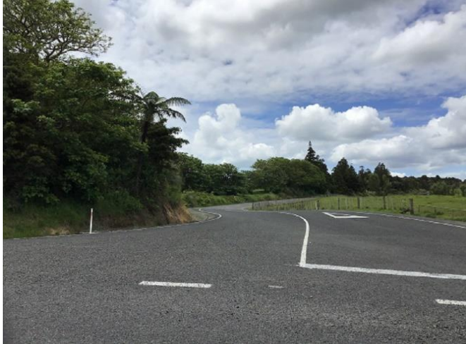
Broadwood Rehab – Completed
