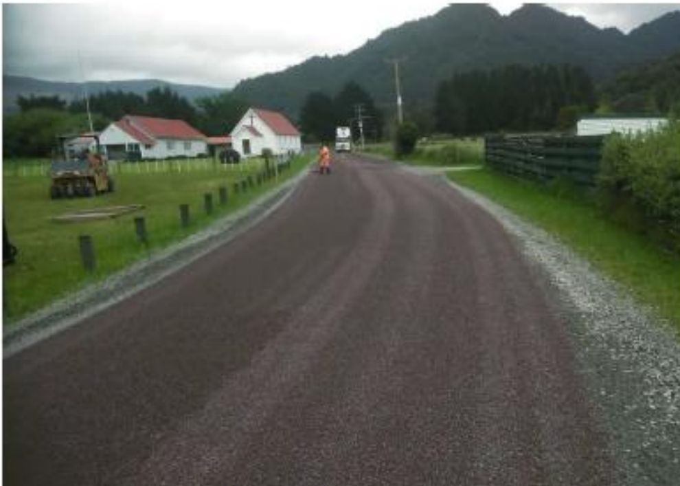
Waima School Rd – Sealed in early November
