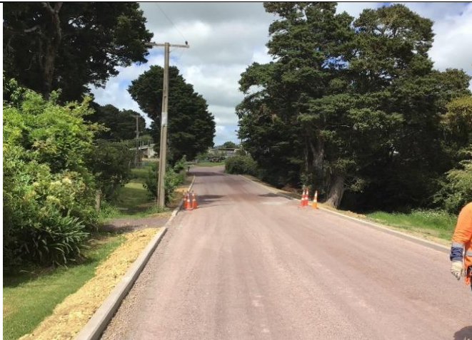
Porotu Seal Extension - Kerb Construction and final trimming
