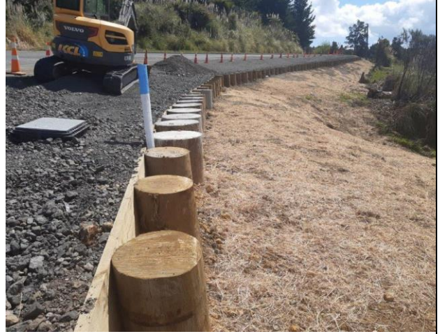
West Coast Road – Timber retaining wall
