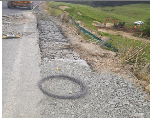
Wainui Road – Gabion shoulder widening and horz drain preparation
