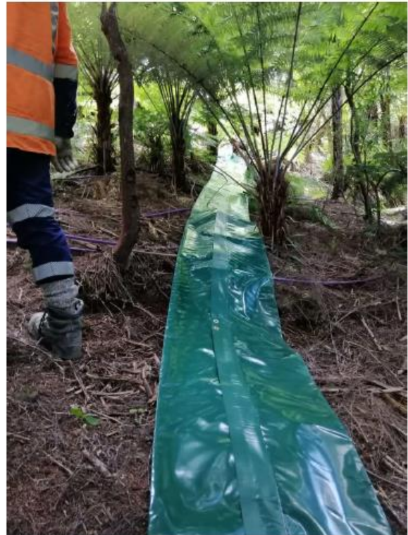
Culvert Sock installed on English Bay Rd
