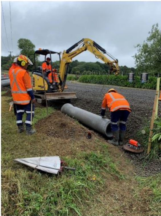
Culvert Installation on Okaihau Rd Rehab
