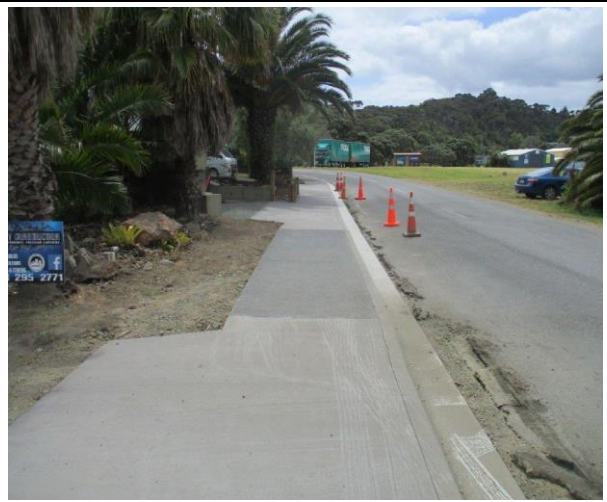
Taipa Point Road – Concrete footpath, kerb and channel
