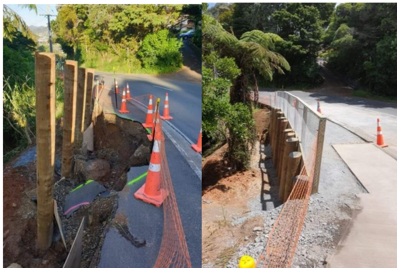
Memorial Dr Footpath Retaining wall
