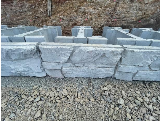
Retaining wall mass blocks
