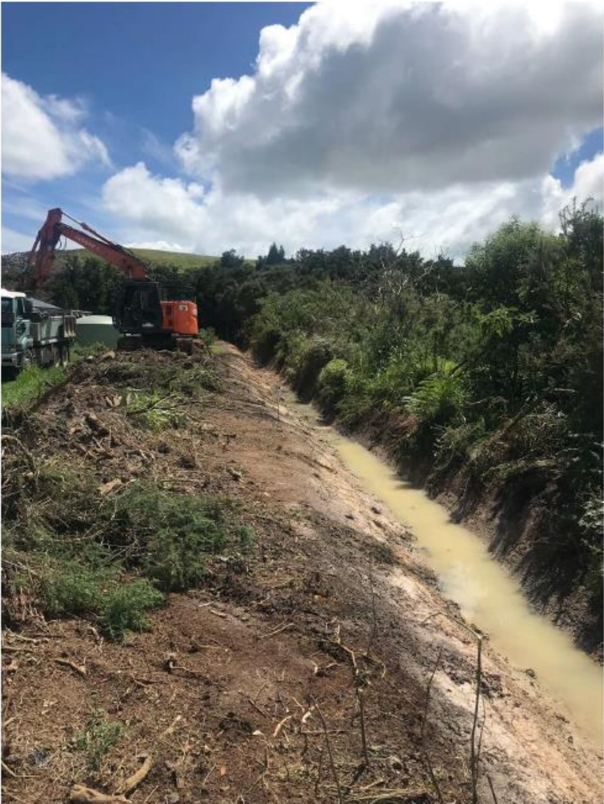
Figure 9: Parapara Toatoa Rd Seal Extension Drainage Works
