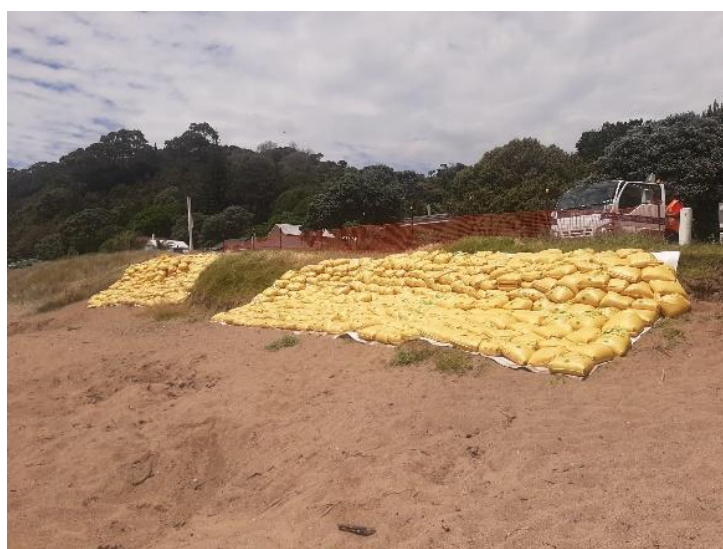
Erosion control work – Long Beach Koiwi Site, Russell
