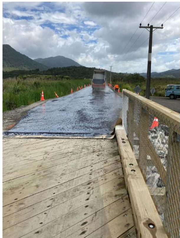
Figure 18: West Coast Rd Bridge Approach
