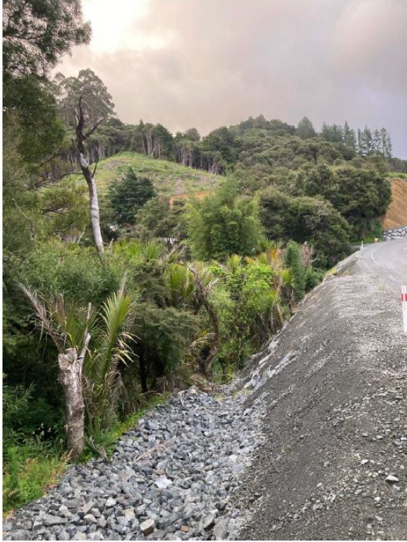
Figure 5: Peria Rd Seal Extension Guardrail Widening
