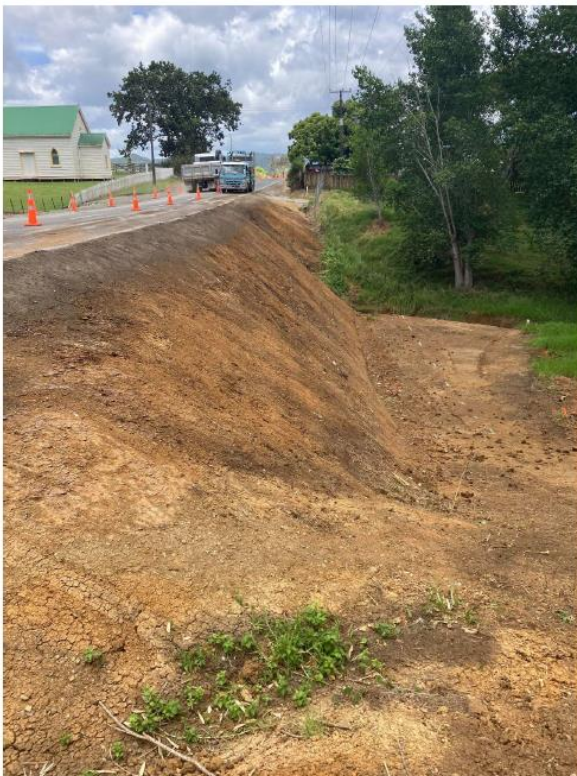
Figure 7: Oruru Rd Rehab 1 Rockwall Preparation
