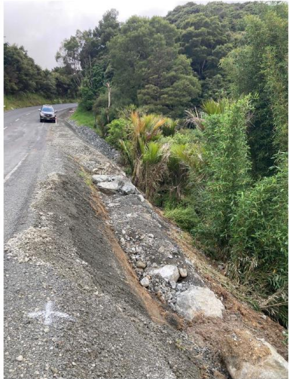
Figure 6: Peria Rd Seal Extension Guardrail Widening
