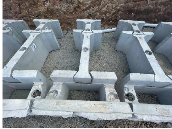
Retaining wall mass blocks
