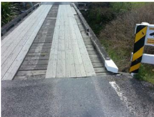
Quarry Rd, Kaikohe – Bridge Repairs to edging and running boards
