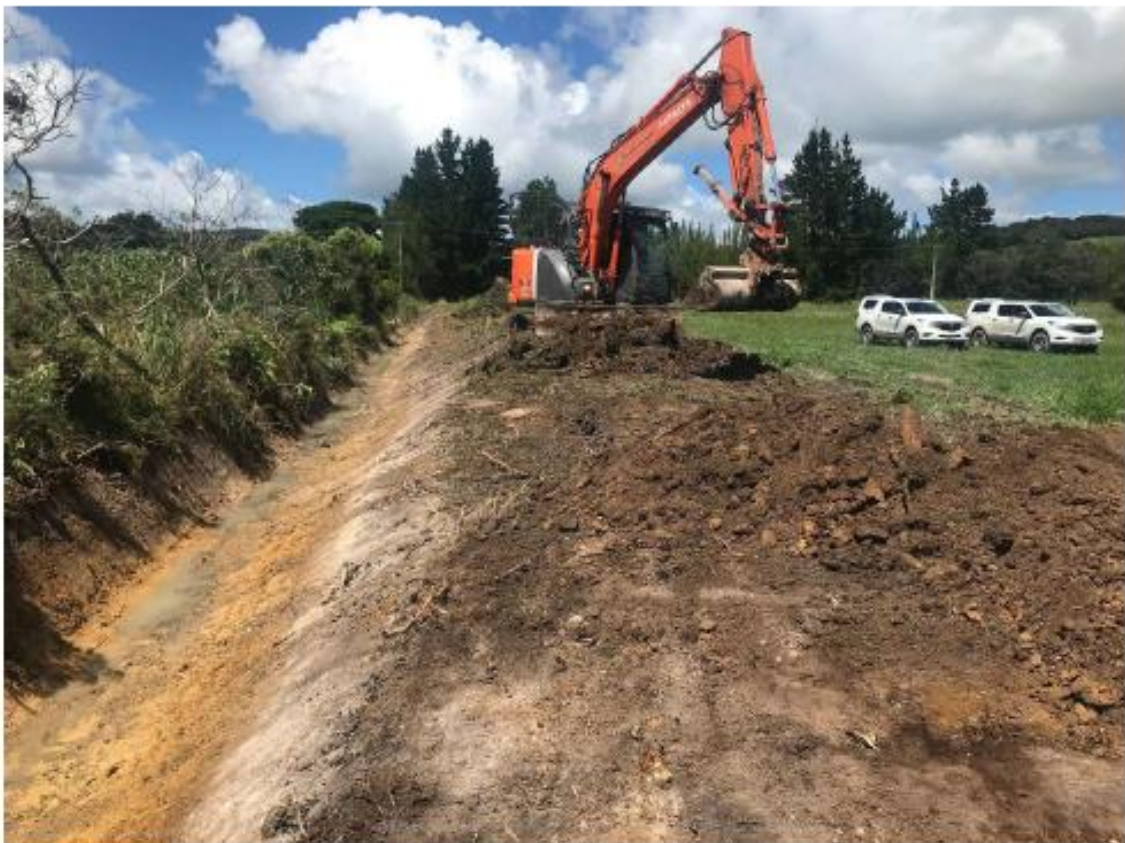
Figure 11: Parapara Toatoa Rd Seal Extension Drainage Works
