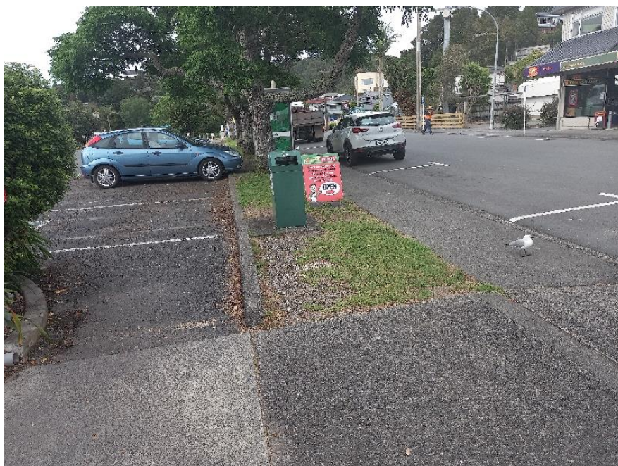
Williams Rd potential trip hazard location
