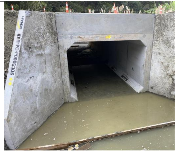
7-23-102 Whangaroa, Waharua & West Coast Road Culvert Renewals - Whangaroa
