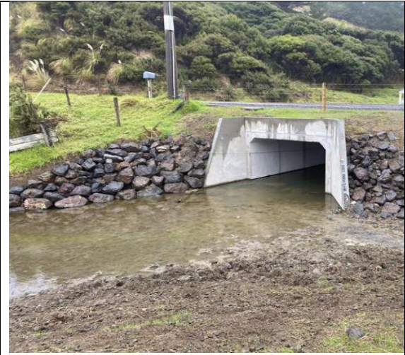
7-23-102 Whangaroa, Waharua & West Coast Road Culvert Renewals - West Coast
