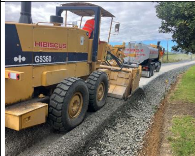
Ruaroa Rd Seal Extension - pavement stabilisation
