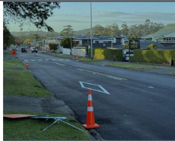
Cobham Road, Kerikeri – Resurfacing (partially complete)
