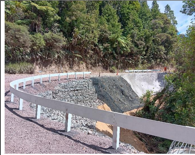
Hupara Road Slip Repair completed
