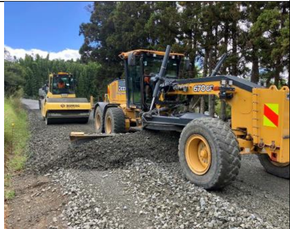
Ruaroa Road Seal Extension - pavement construction
