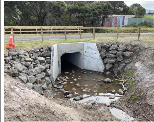
7-23-102 Whangaroa, Waharua & West Coast Road Culvert Renewals - Waharua
