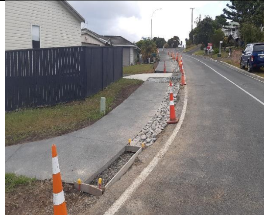
Cable Bay Block Road - Preparing for pedestrian crossing.
