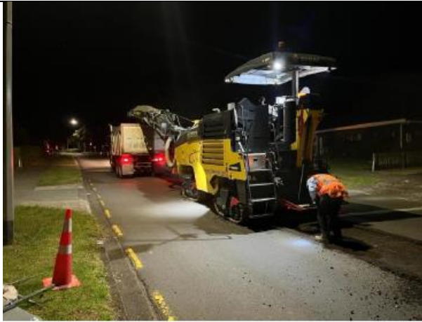
Cobham Road, Kerikeri – Resurfacing (night works).
