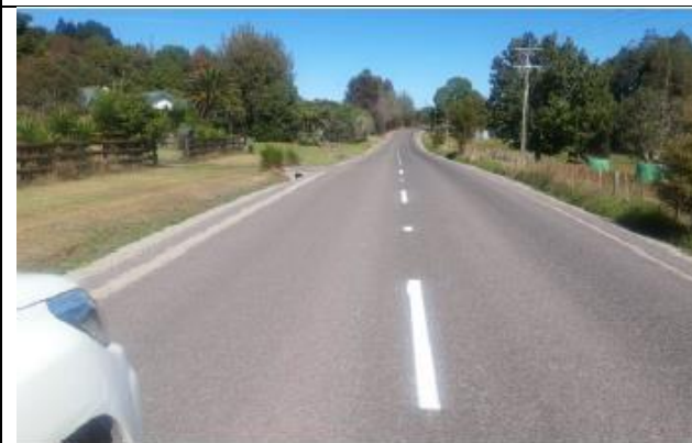
Cumber Road Rehabilitation
