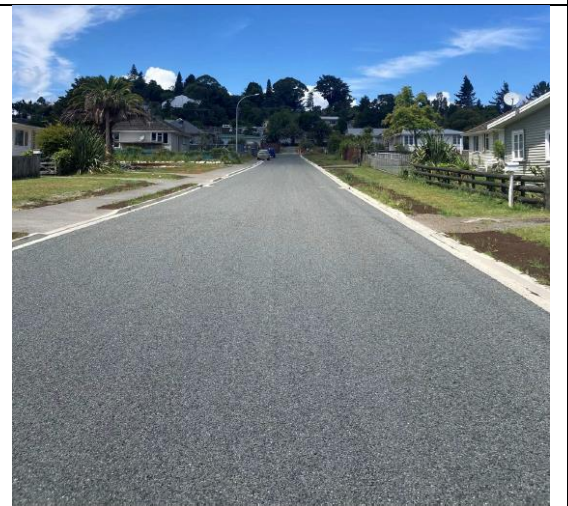
Sommerville Ave, Kaitaia - Rehabilitation and replacement of failed stormwater reticulation (completed).
