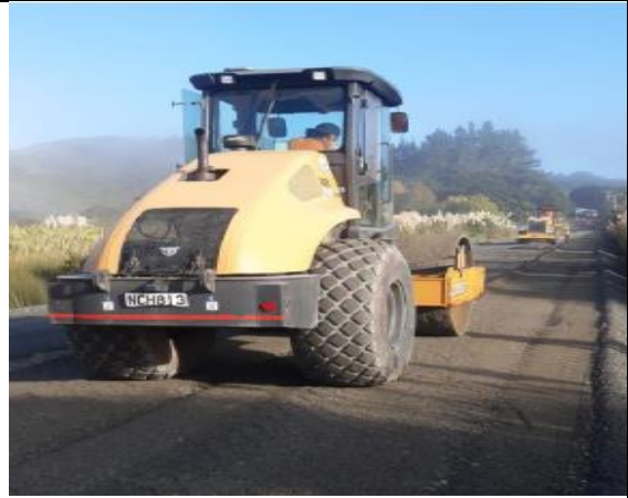
Paroa Bay Road, Russell - resurfacing, including a section of rehabilitation.
