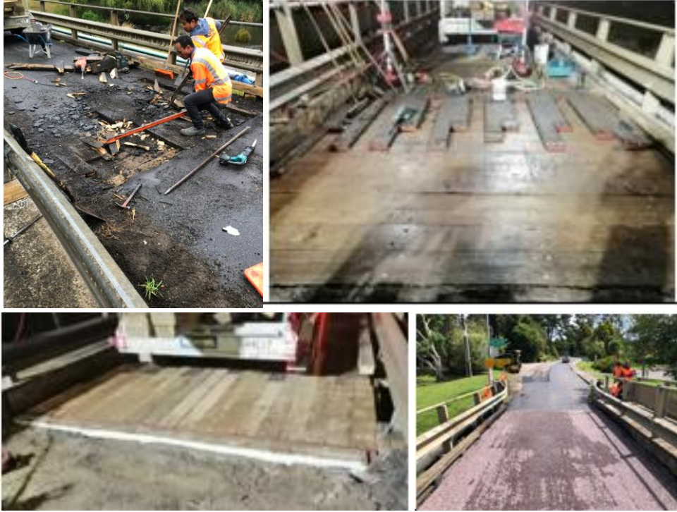
7/21/214 General Bridge Repair (SP3) - Landing Road Bridge S09
