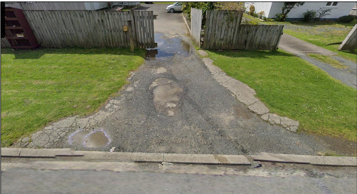
Figure 2: Existing Vehicle Crossing to be upgraded.
