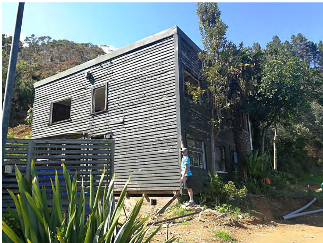
Figure 5: Possibly the last building of the WWII army camp (Rochelle Jacobs 2017).
