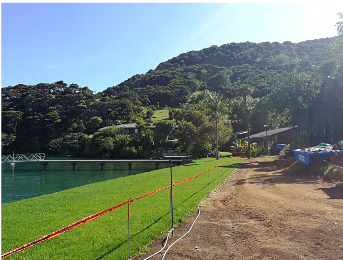
Figure 7: Further earthworks close to the lodge buildings. (2017).
