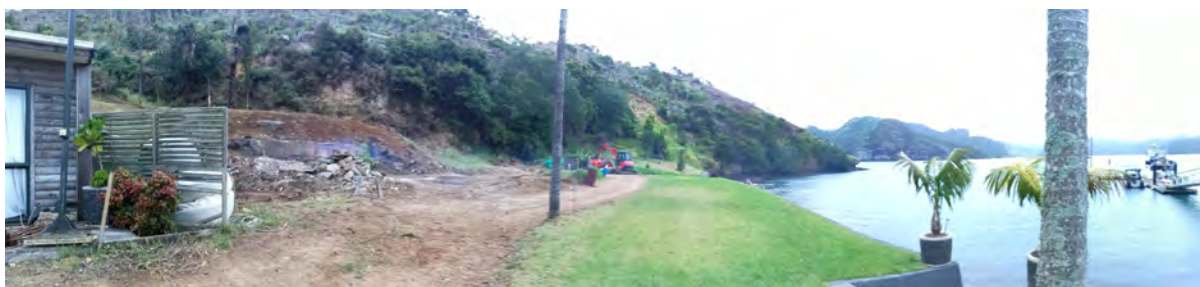
Figure 6: Demolition of the building (2018).
