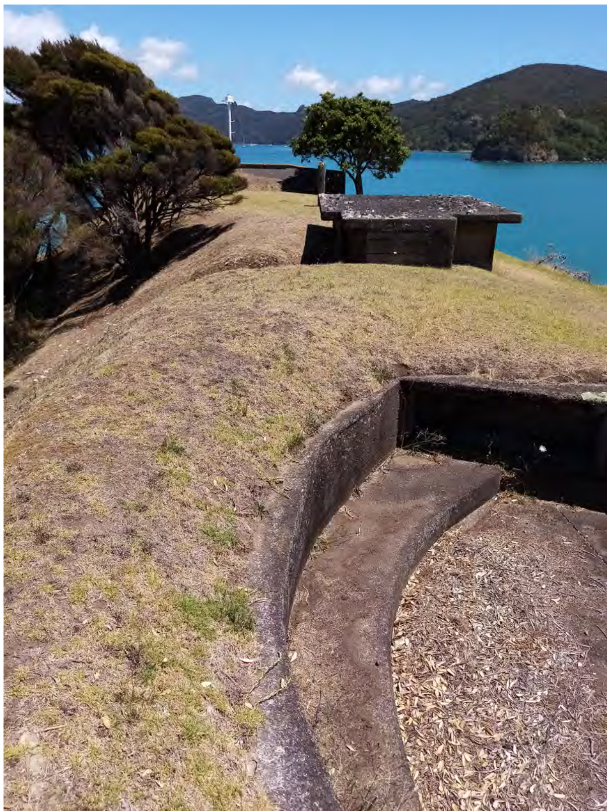
Figure 18: Gun emplacement structures.
