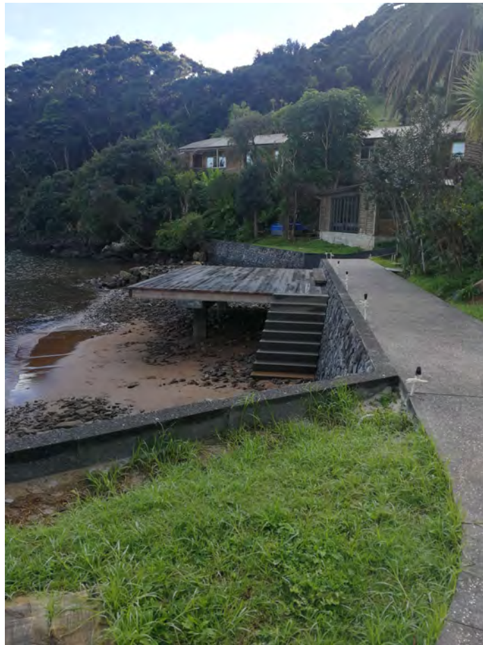
Figure 8: Further building works in 2019.
