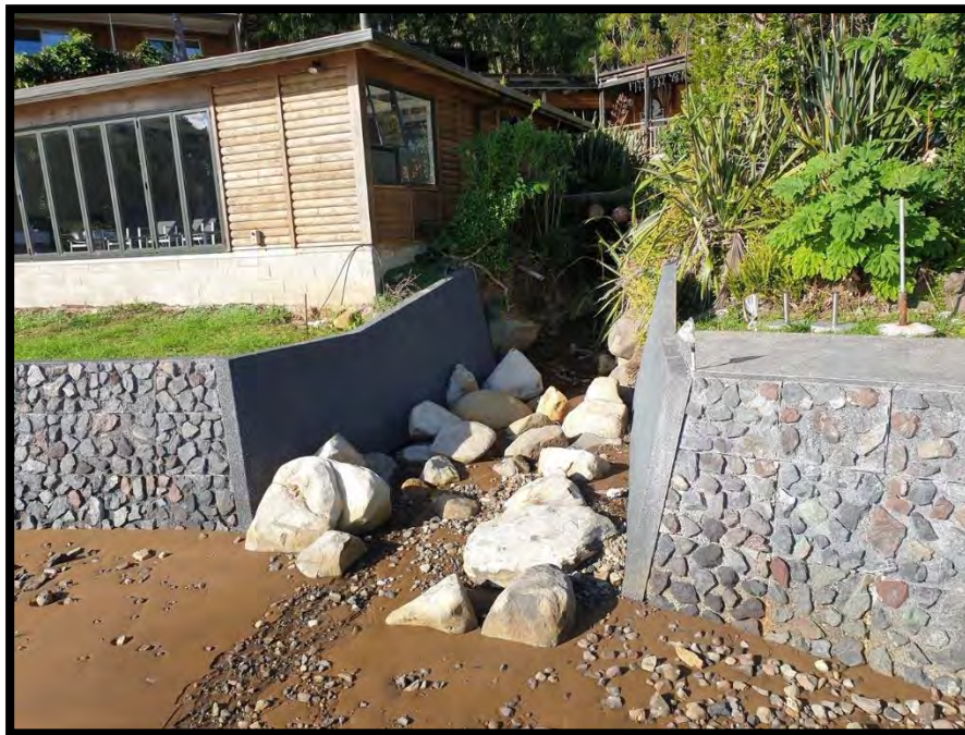
Figure 4 - Existing stream and seawall (photo date - May 9 2021)
