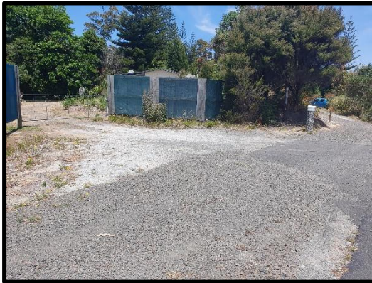
Figure 24: Existing southern vehicle crossing.
