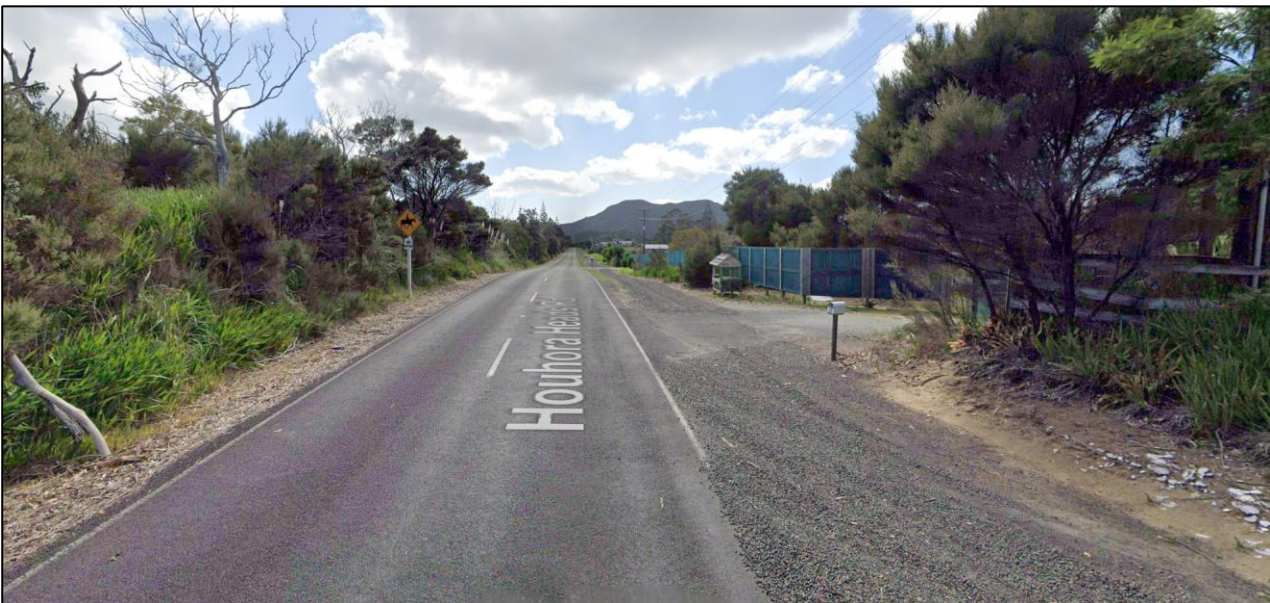
Figure 13: View of existing southern access point on Houhora Heads Road facing northeast, >170m sight distance available along southbound lane.
