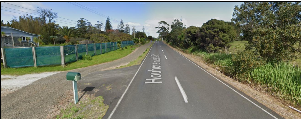
Figure 16: View of existing northern access point on Houhora Heads Road facing southwest, estimated 138m sight distance available due to local high-point obstruction.
