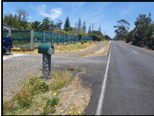
Figure 30: Views along the northbound lane, taken from the northern crossing. The middle crossing can be seen in the distance and the crest of the hill which obstructs the required SSD.
