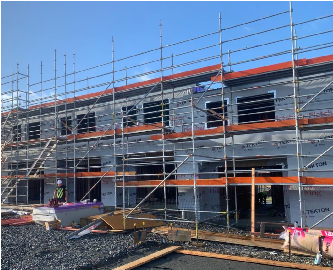
Figure 8 Photograph of a scaffold with buttress bay, credit: Wain Chambers
