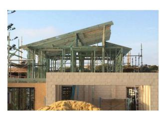
Wall framing comprises studs, top plates, bottom plates, and lintels.
