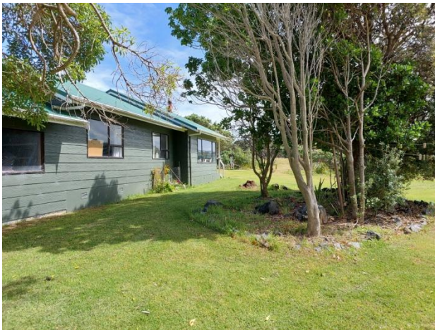
East side of existing house
