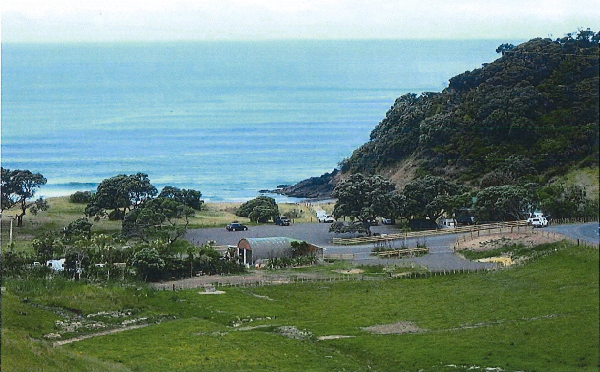
Photo 3: Overview of the project site, a work in progress: Access off Rawhiti Road recontoured and sealed, new site managers' house site prepared at lower right, day visitor parking area currently presenting somewhat utilitarian appearance with inadequate capacity for expected visitor numbers, and wide timber boardwalk and dune fencing guiding low-impact access to the southern end of the bay.
