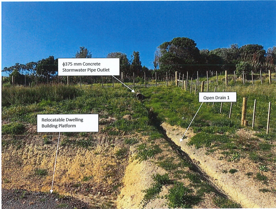
Figure 6. Existing Stormwater Pipe Outlet
