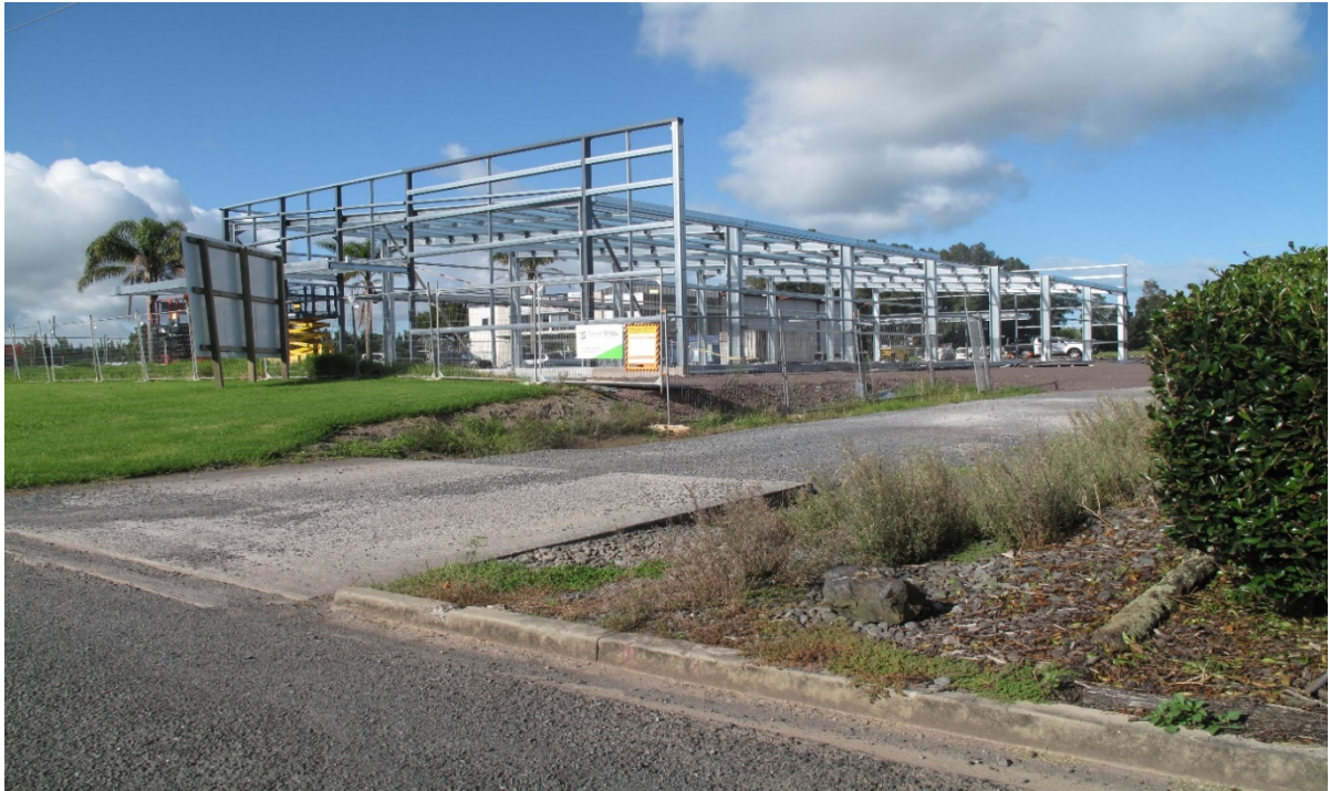
Above photo of New Commercial building under construction depicting raised building platform in Klinac Lane. Photo's taken February 2023
