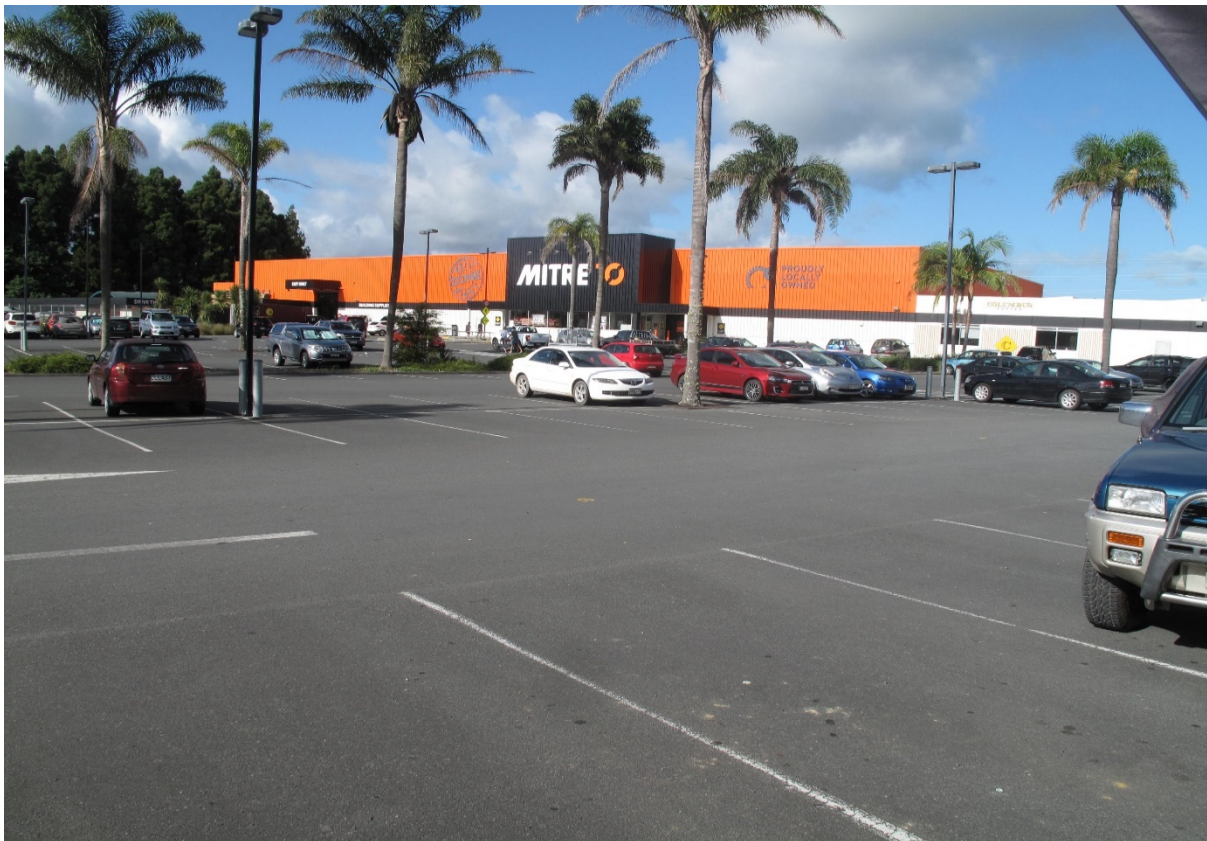
Lower Photo featuring extensive sealed parking areas that is common to the entire Waipapa commercial and industrial centre.
