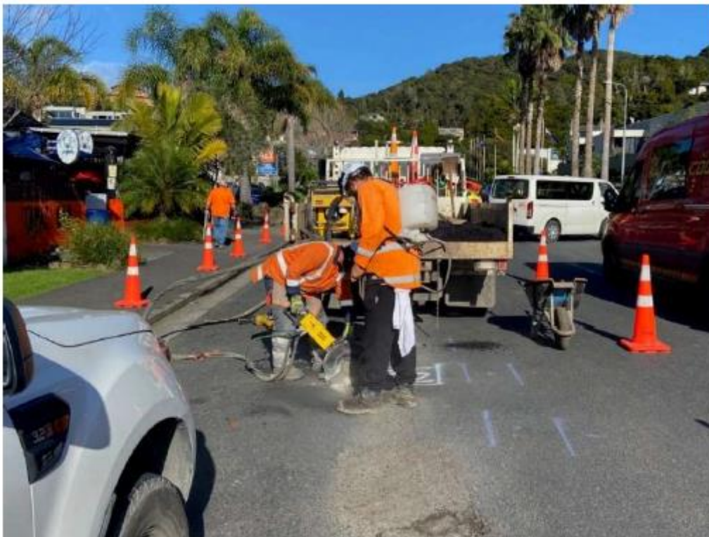
Figure 12 - Kings Road - Test Pit Investigations
