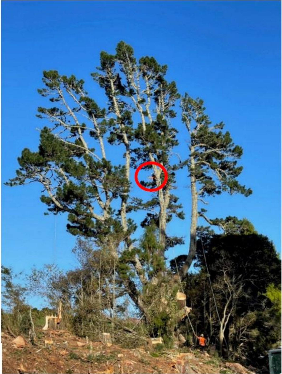
Figure 5 - Puketotara Rd - Tree Removal (Where's Wally)
