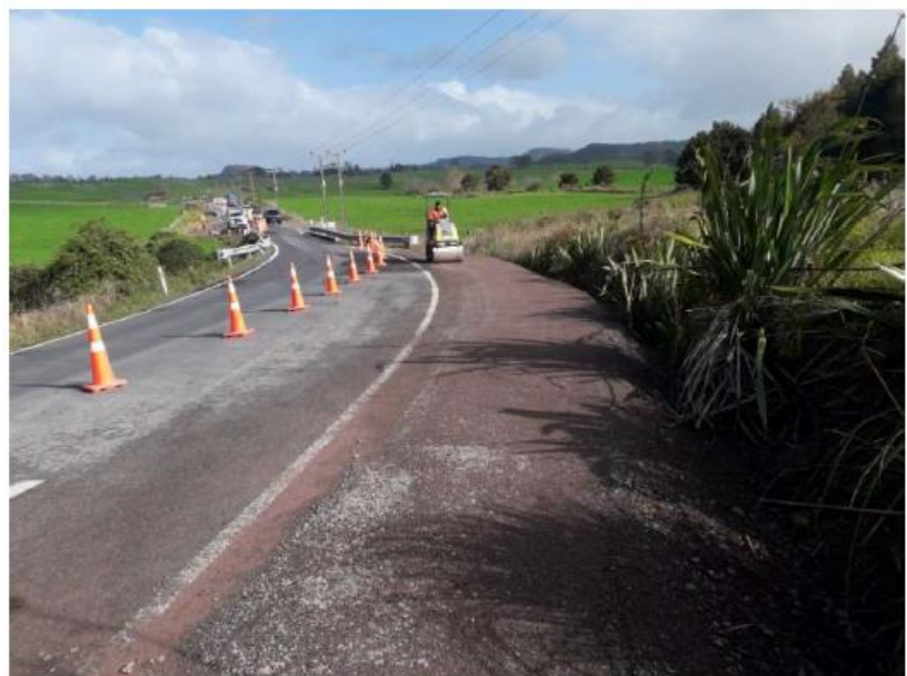
Figure 14 - Old Bay Road - Shoulder Widening Prep for new Guardrail
