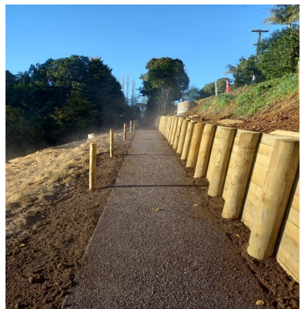
Pa road Footpath showing retaining wall section
