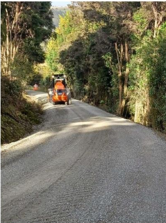
Figure 11 - Waikino Road & Pokapu Road - Heavy Metalling
