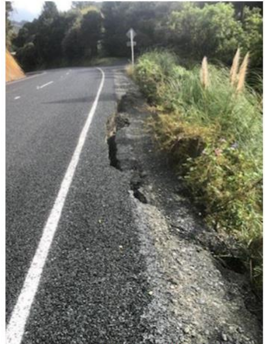
Figure 2: Section Four Underslip
