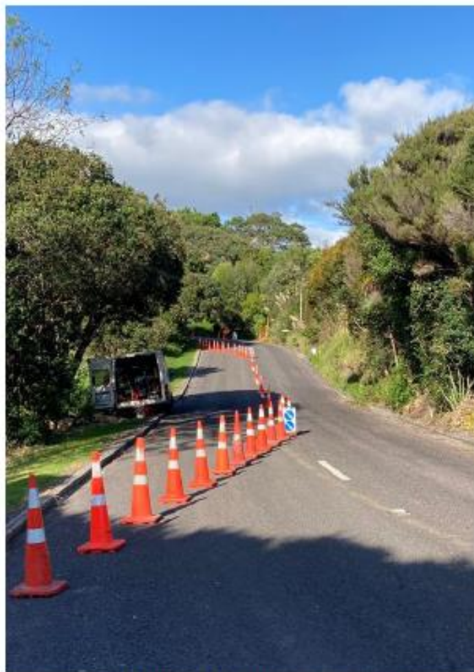
Figure 6: Powells Road CCTV prior to drainage works
