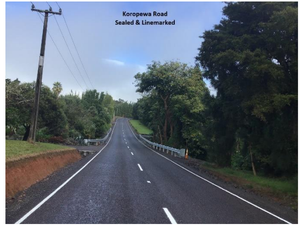
Koropewa Road/Sealed and line marked
