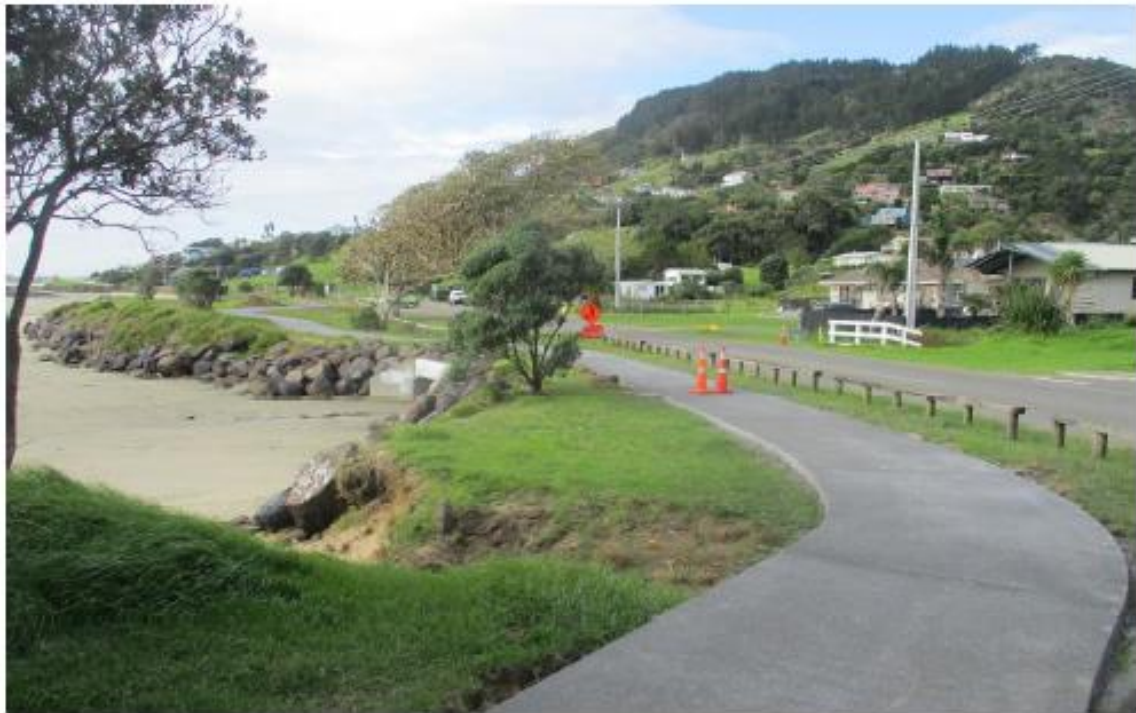
Figure 5: Foreshore Rd Ahipara New Footpath
