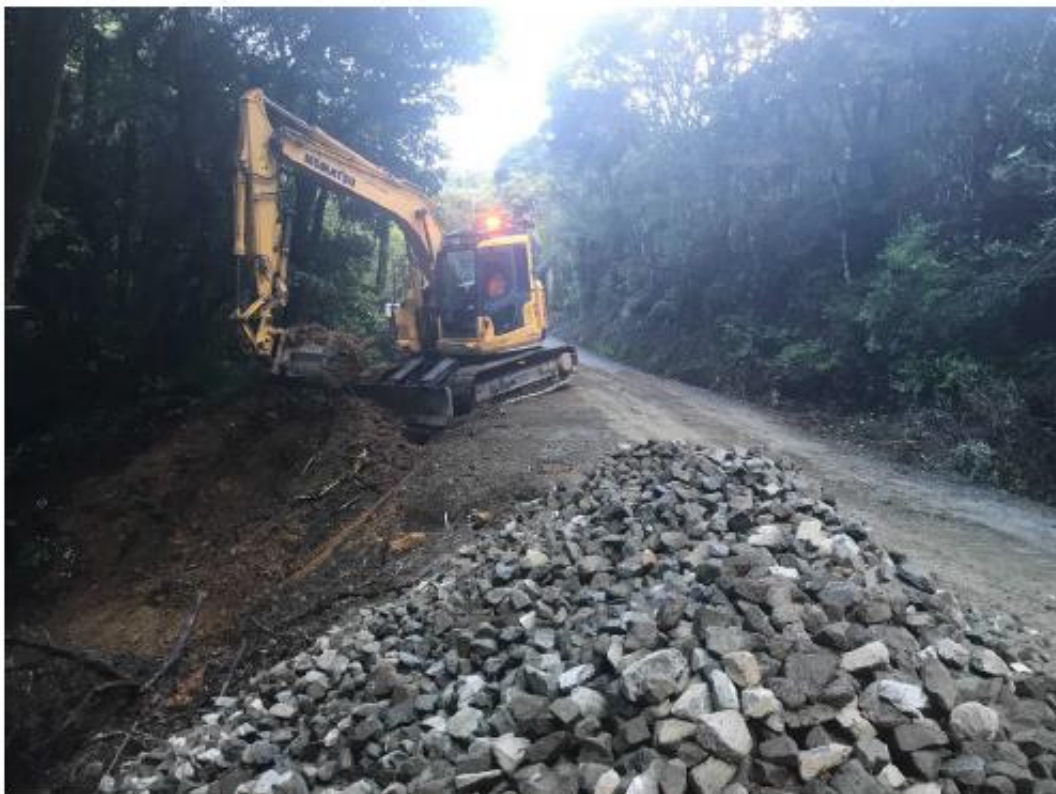
Figure 8: Diggers Valley Culvert Replacement in progress
