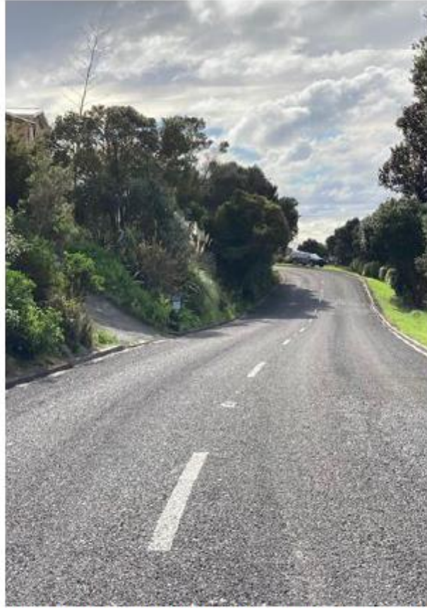
Figure 7: Powells Rd Pavement Reinstatement / Levelling after drainage repairs
