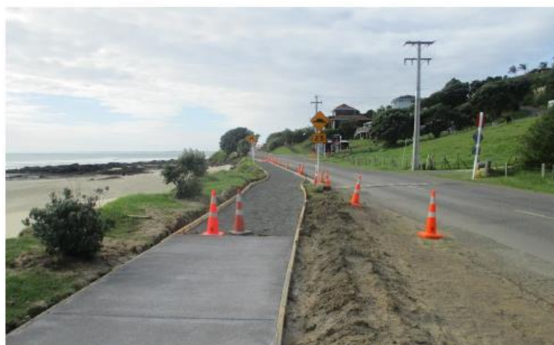
Figure 4: Foreshore Rd Ahipara New Footpath
