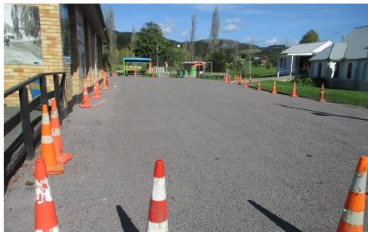
Figure 3: Kaeo Carpark Repairs
