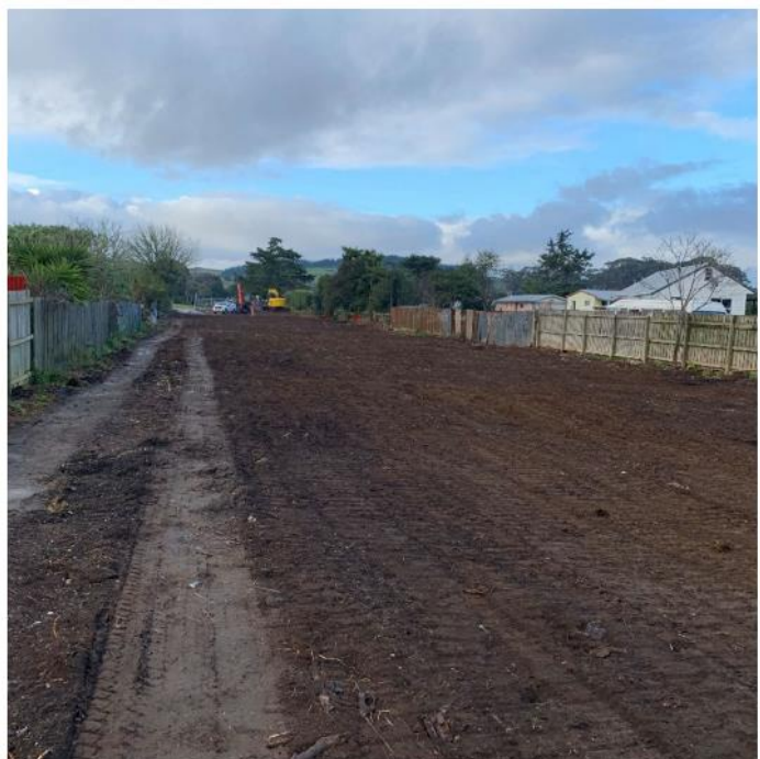
Figure 13 - Moerewa Paper Road Clearing of Asbestos
