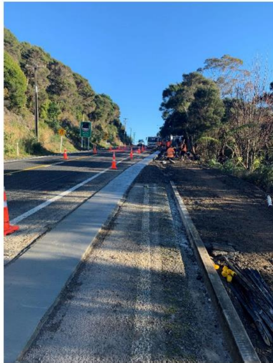
Figure 8 - SH11 Haruru - Minor Safety Improvements
