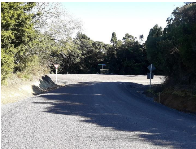
Pungaere Road / Waiare Road Intersection Rehab
