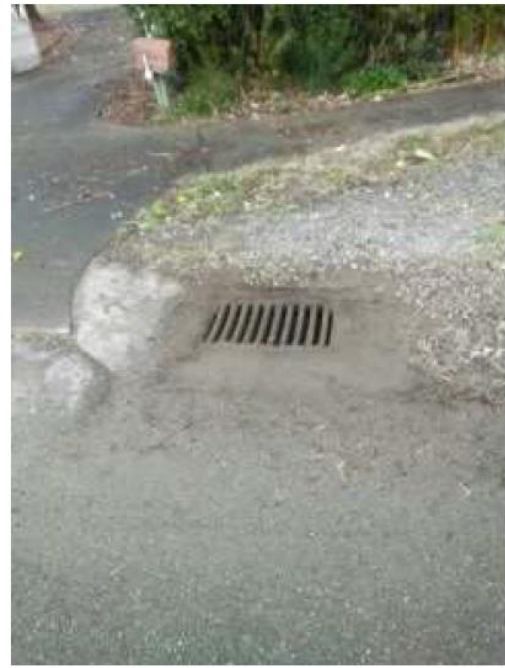
Figure 4 - Grate Clearing - Before and After
