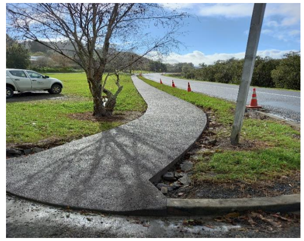
Kohukohu Road Footpath
