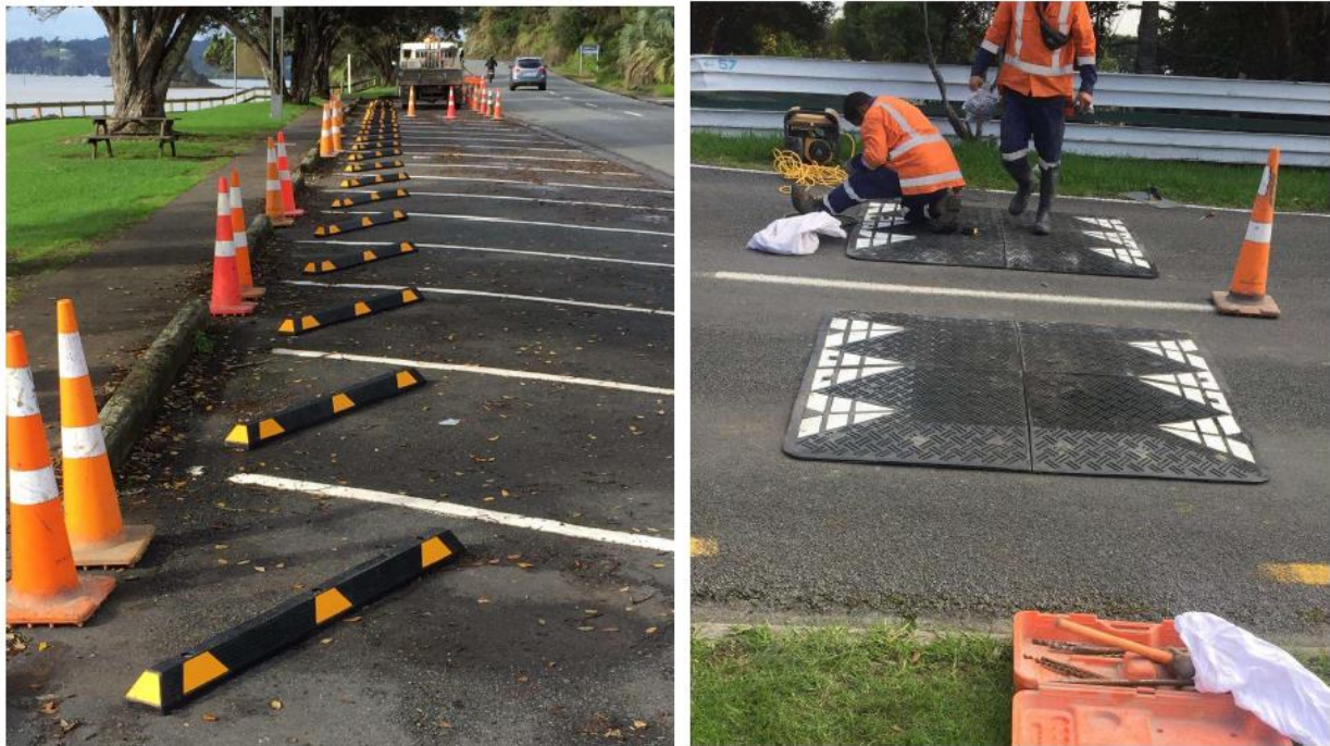
Figure 6 - Rawene Speed Cushion Installation & Paihia Wheel Stops
