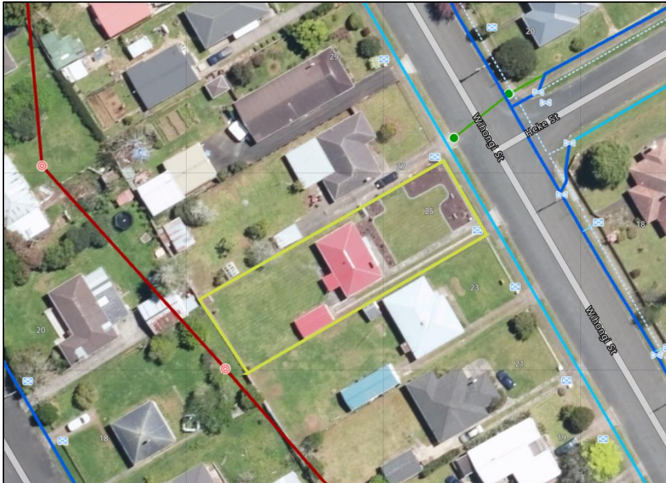
Figure 1 – Aerial view of the development site, taken from Far North District Council 3 Waters Maps
