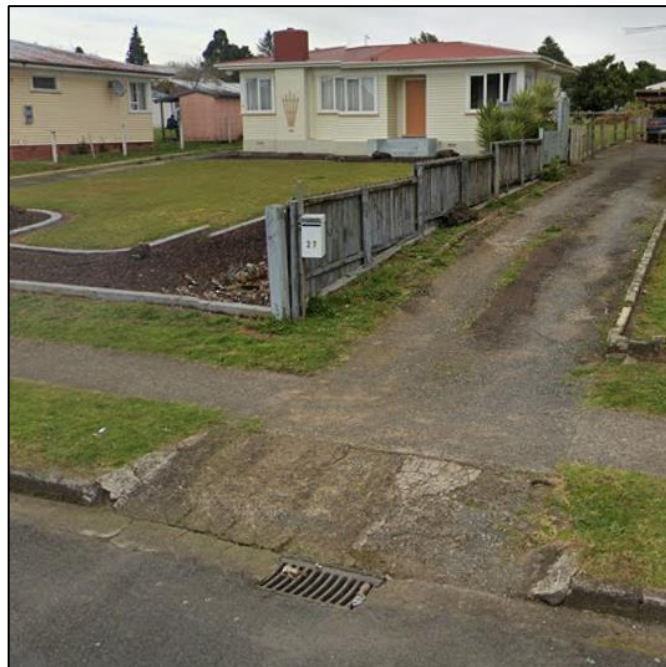
Figure 4 – Existing public stormwater catchpit located at the end of the vehicle crossing of 27 Wihongi Street.
