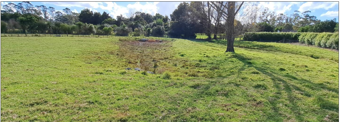
Figure 3: Site Photograph of the Detention Pond, Taken on the Day of the WJL Fieldwork Investigation (22.05.2024) - (northwest direction)
