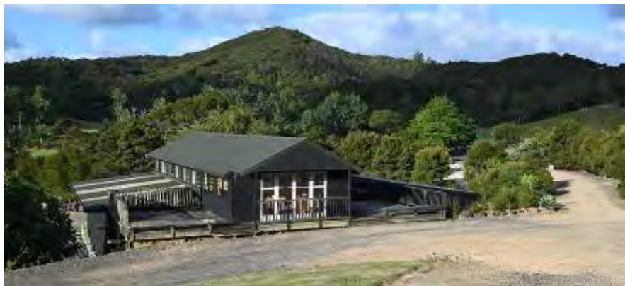
Photograph 13: The building that is intended to be utilised as a community facility. Its basement would continue its current role as a workshop and for equipment storage.
