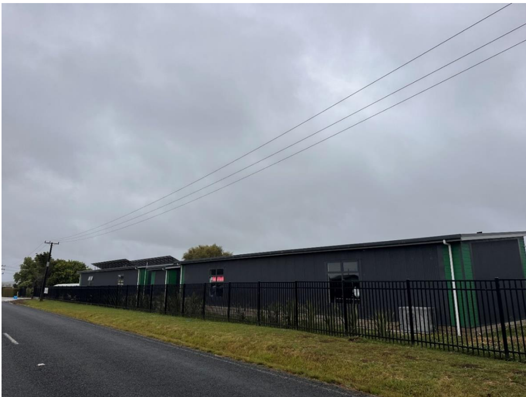
The photo above shows the existing Kura buildings consented under RC 2220673.
