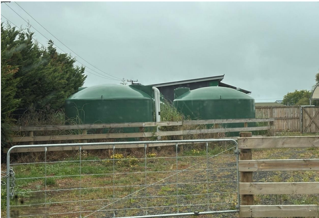
The photos above show the existing water tanks that are utilised for fire fighting water detention and attenuation for the Kura, as detailed within the stormwater report approved under RC 2220673.
