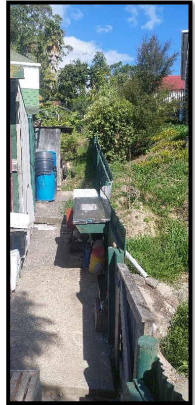
Figure 12 - Location of sunlight infringement with landscape retaining wall in background
