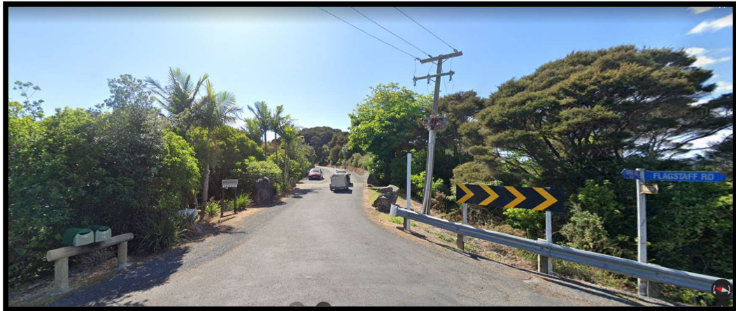
Photograph 1: Pukematu Lane showing sealing and powerlines
