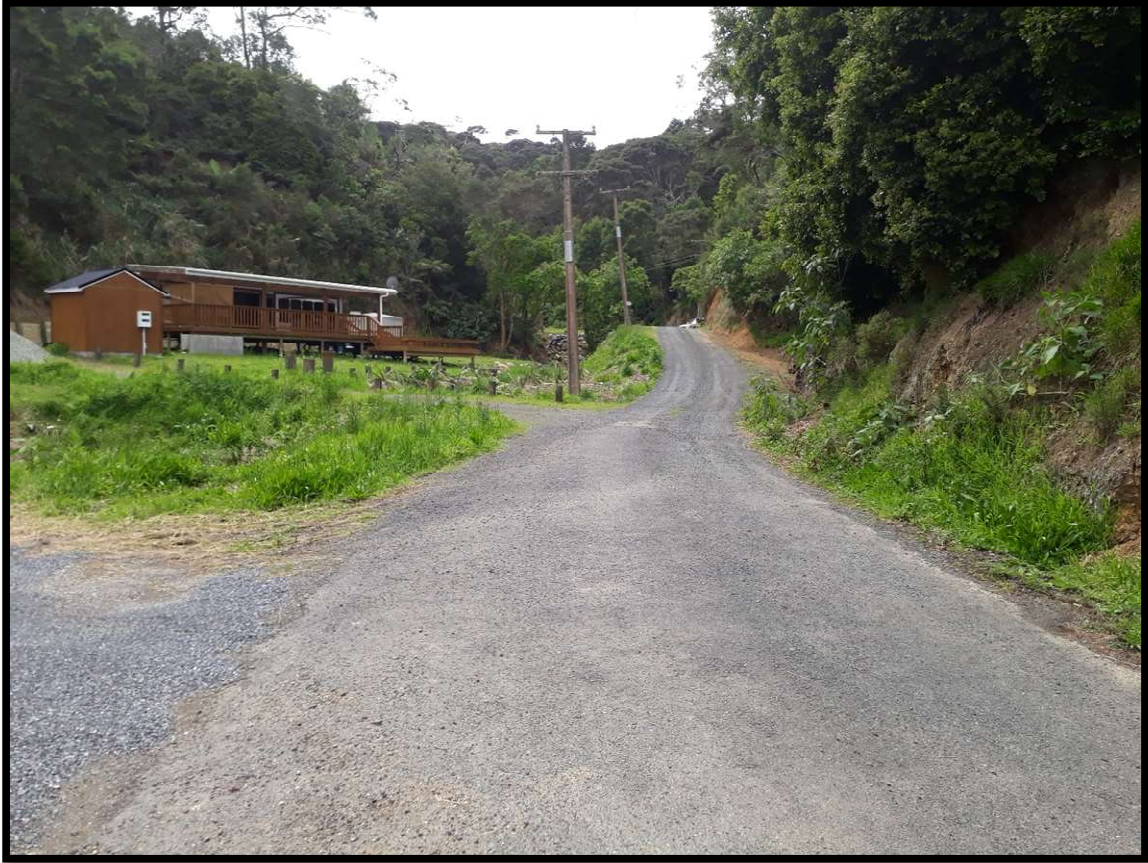
Photograph B4: Start of metal driveway up to 24 James Street (18 James Street on the left)
