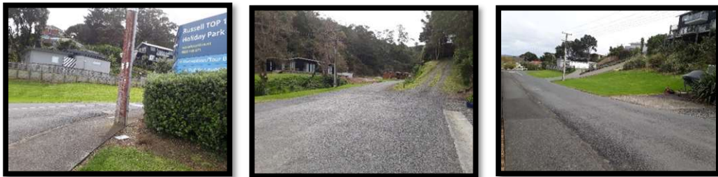
Photographs 2 – 4: James Street showing extent of sealing and powerlines
