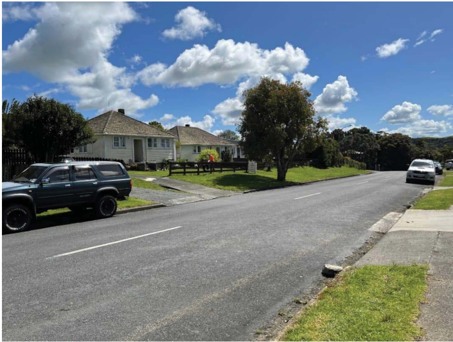
Photograph Appendix A.10: Worth Street (looking north) showing the driveways of Nos 7 and 9. Photo taken from opposite 9 Worth St
