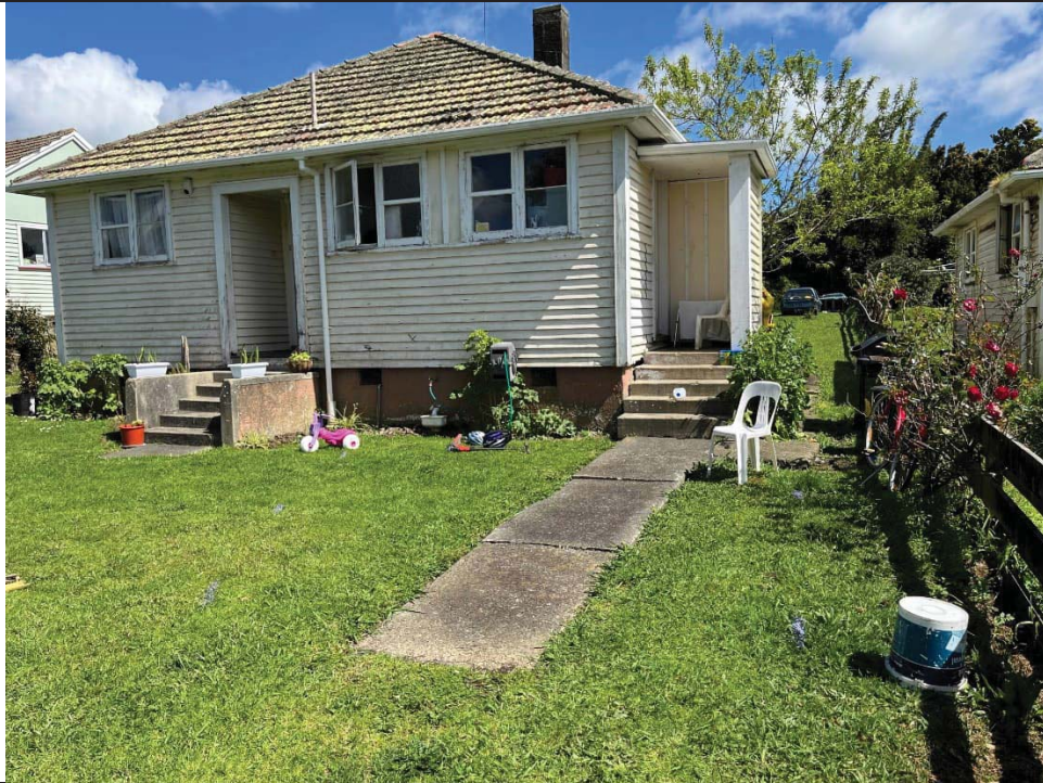
Photograph Appendix A.5: Front of dwelling of 7 Worth Street (looking northwest)
