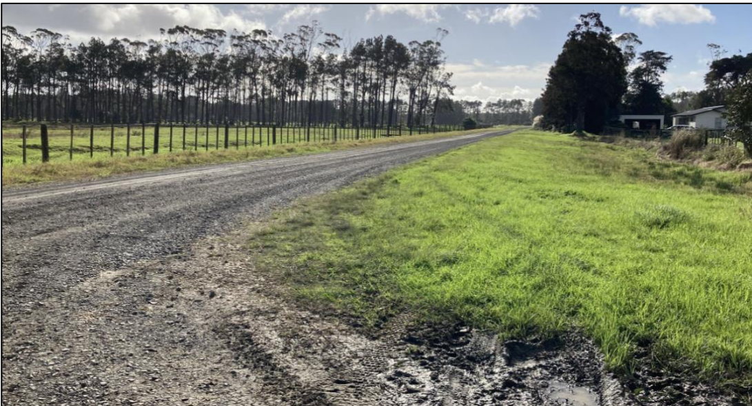
Figure 5: Sighting Distance looking North
