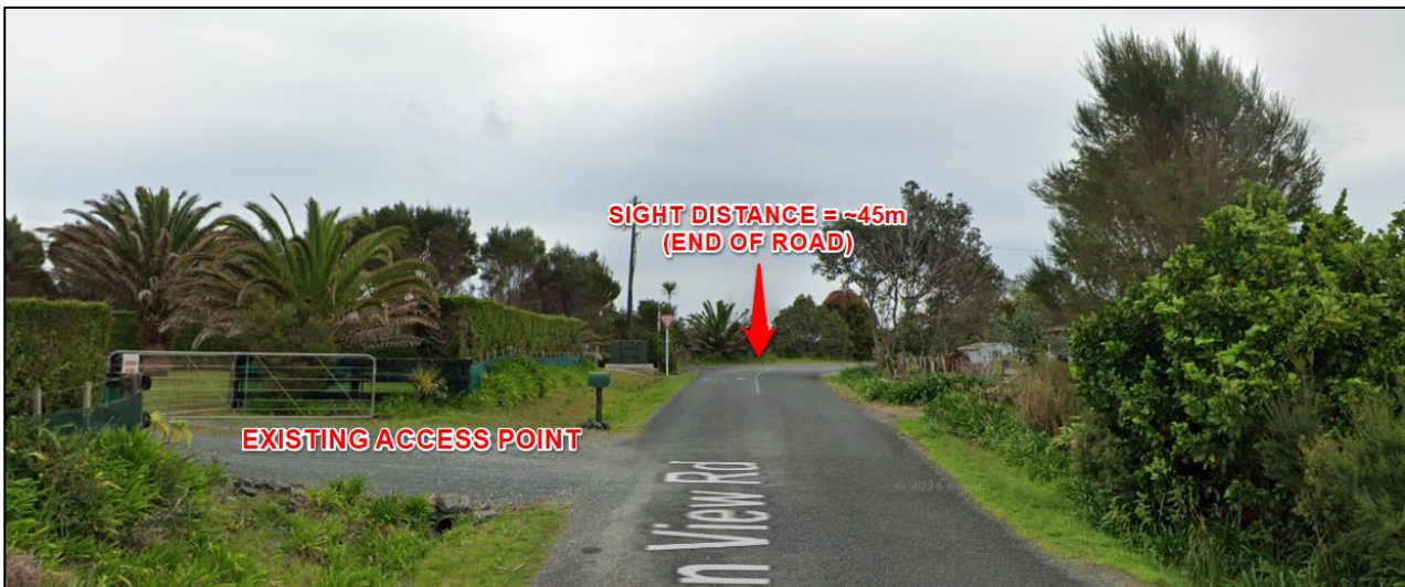
Figure 8: Existing Access Point on Ocean View Road Facing West, ~45m Sight Distance Available to End of Street.
