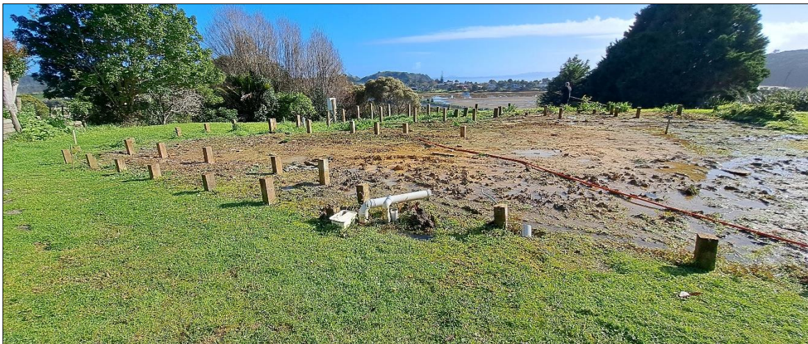
Figure 4: Site photograph (Northwest direction) overlooking Proposed Building Platform.
