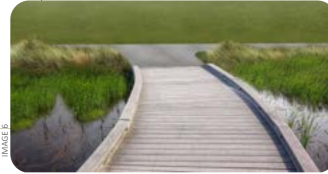
BRIDGE OVER SMALL PERPETUAL WATERCOURSE
