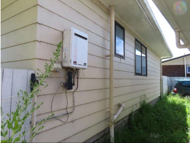
Right of rear elevation
