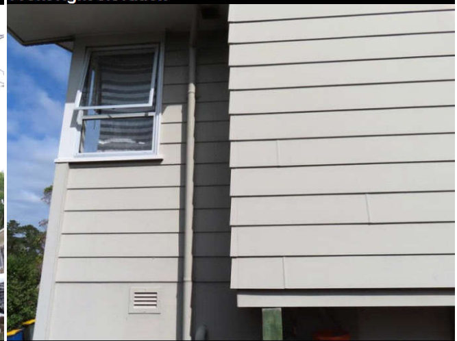
Right of rear elevation
