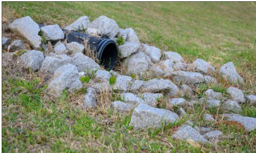
Figure 7: Typical Riprap Outlet
