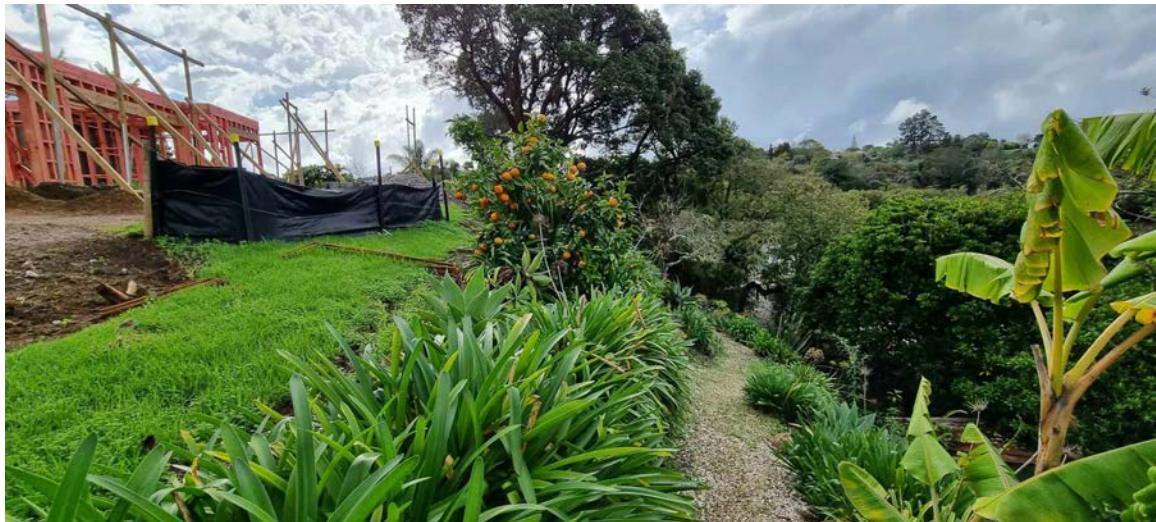
Figure 4: View from the southern side of the reserve (Lot 3 DP 87102) below house site
