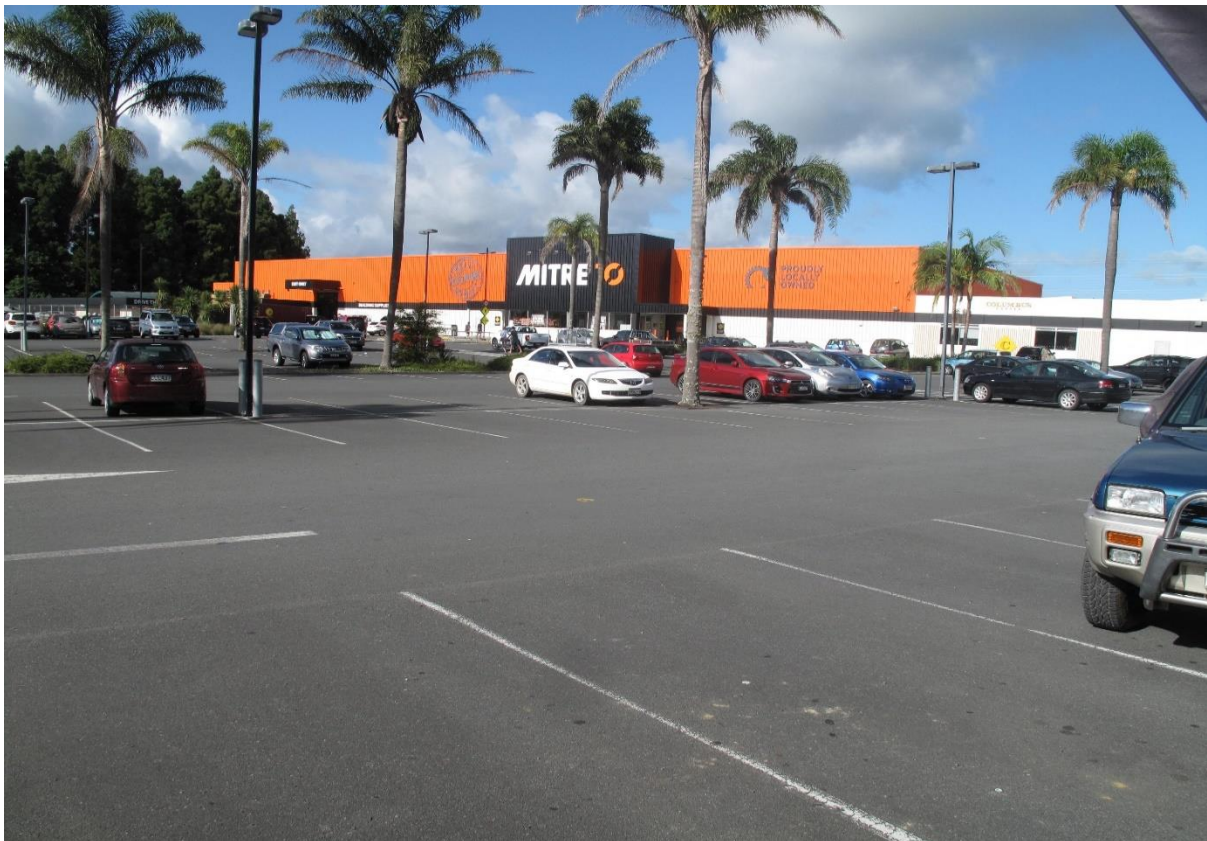
Lower Photo featuring extensive sealed parking areas that is common to the entire Waipapa commercial and industrial centre.
