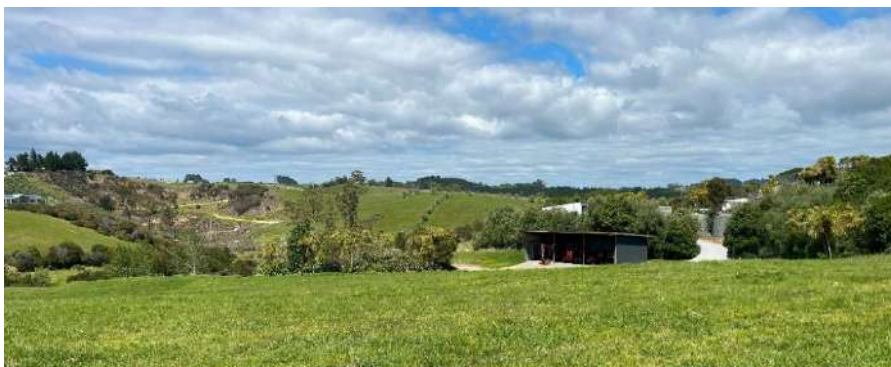
Photograph 1: Looking west over existing built development within Lot 1.
