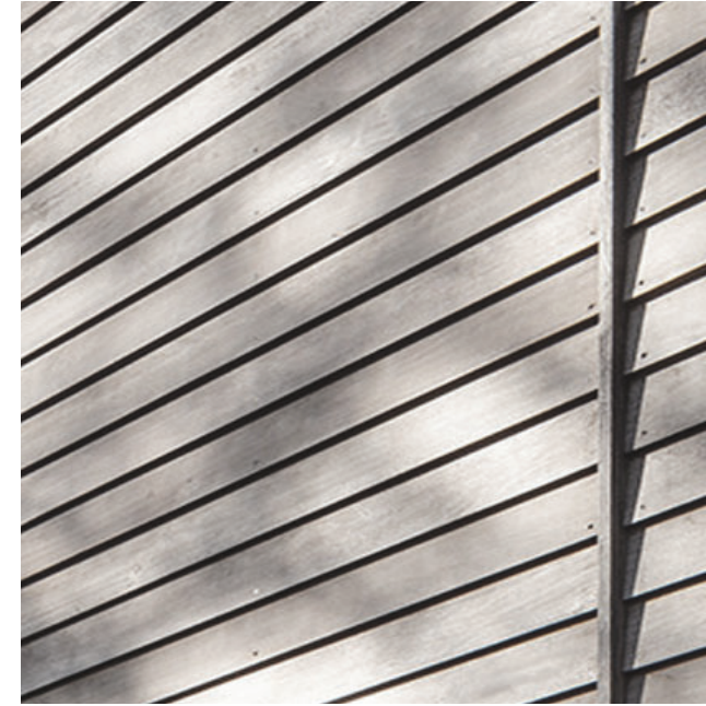
3 EXTERIOR WALLS + CLADDING
