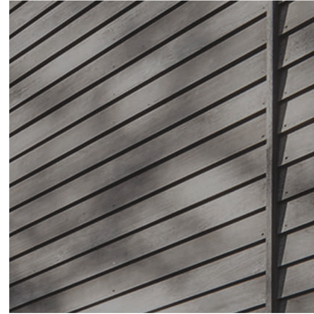
3 EXTERIOR WALLS + CLADDING
