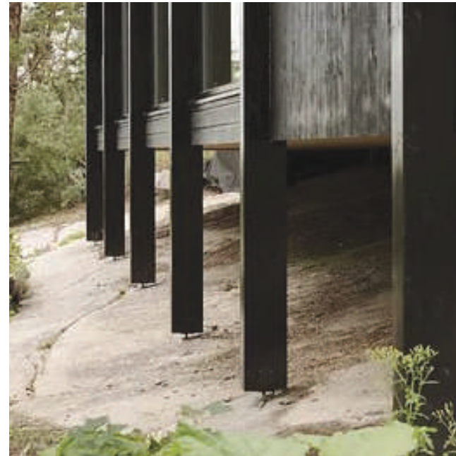
5 EXPOSED STRUCTURAL FOUNDATIONS
