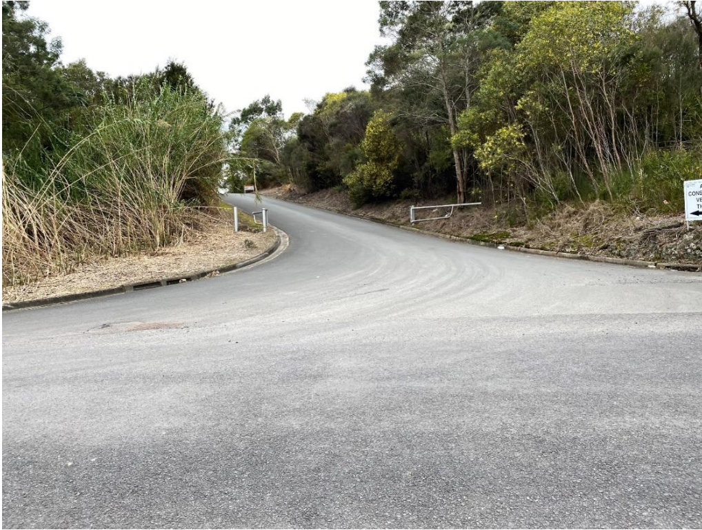
Figure 2 - Entrance to Hospital Road from Greenacres Drive
