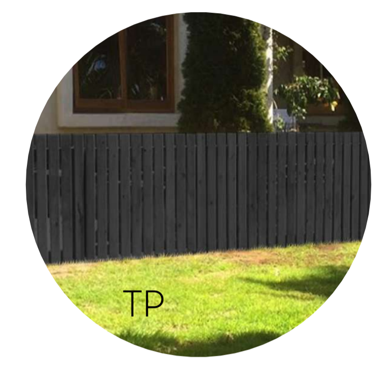
1.2m Timber paling fence
