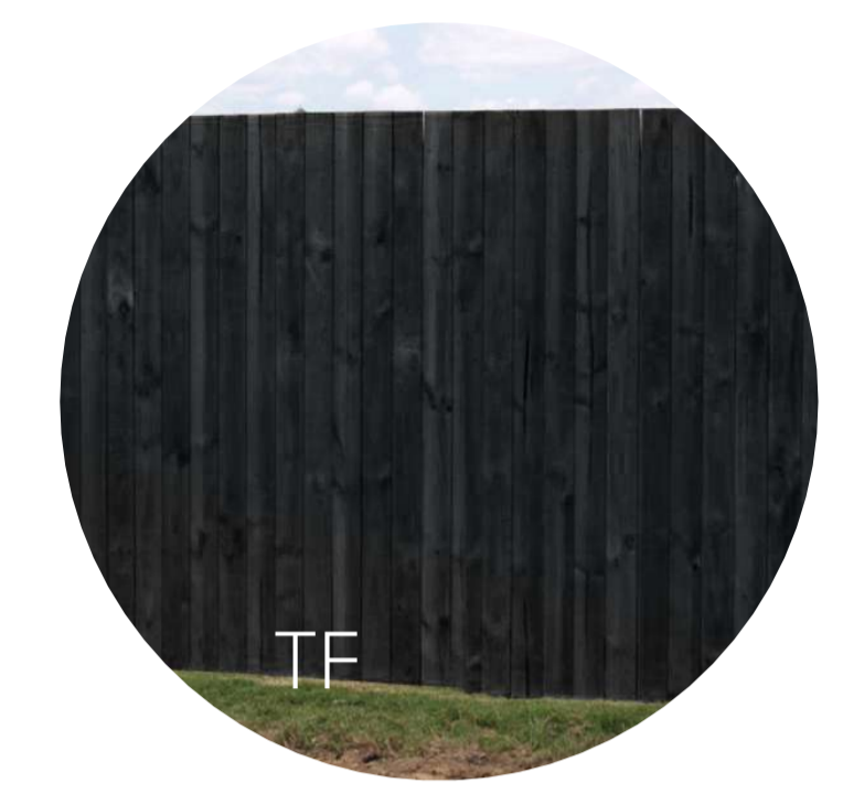
1.8m Timber paling fence
