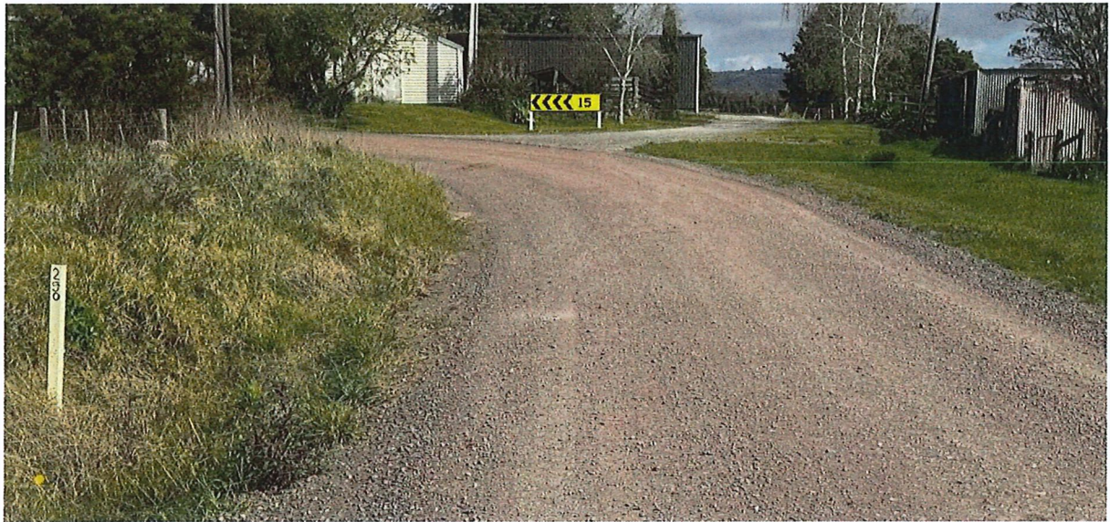
Photo 5. Looking east along Okokako Road from 230 metres. The width for 1.5 kilometres beyond this point is between 4.2 and 4.8 metres.
