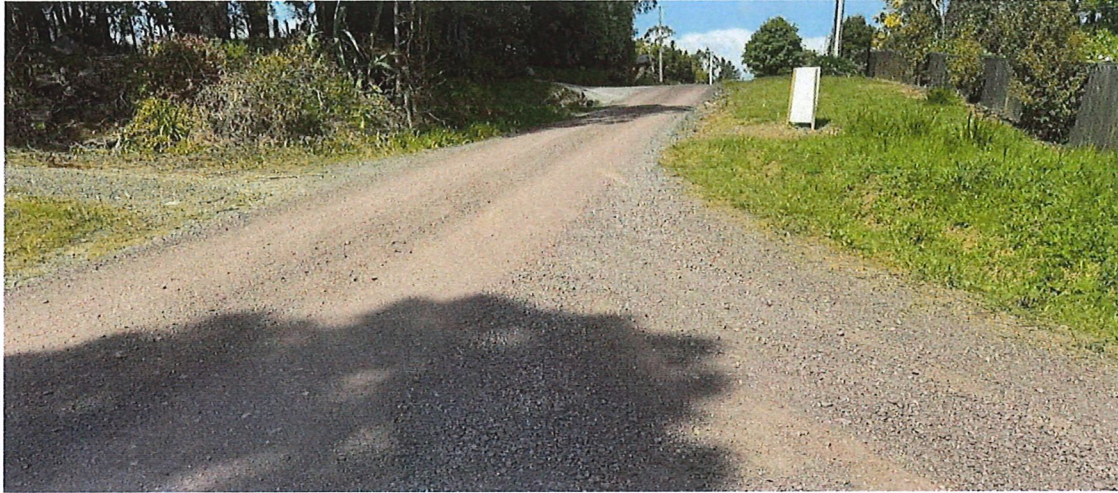
Photo 11. Looking north along Okokako Road from 2340 metres. The forward visibility over this crest is adequate for the expected operating speeds of 35 km/hr.
