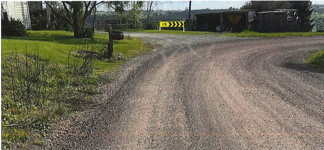
Photo 3. Looking north along Okokako Road from 200 metres including the proposed chevron warning sign. Space is available for this within road reserve and clear of driveways and buildings. Widening is also proposed through the bend as per Figure 1.
