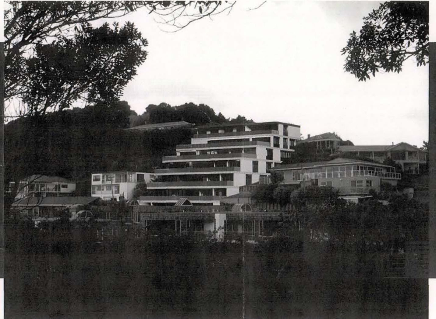
NORTH WEST VIEW FROM SHORE LOOKOUT
