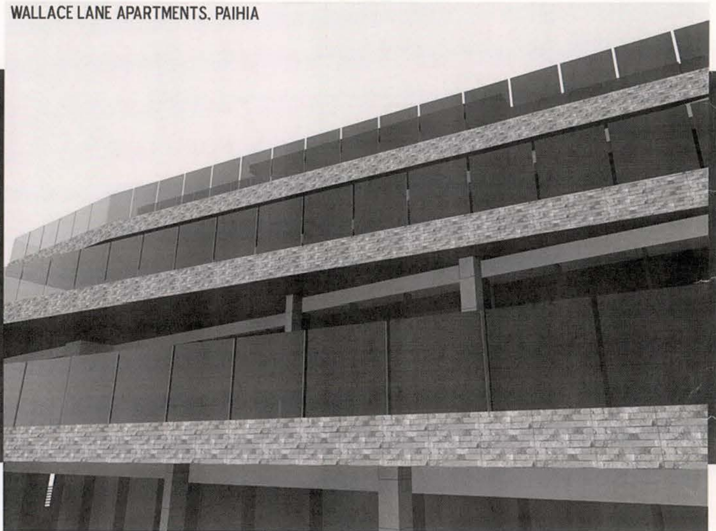
VIEW LOOKING TOWARDS TOP
