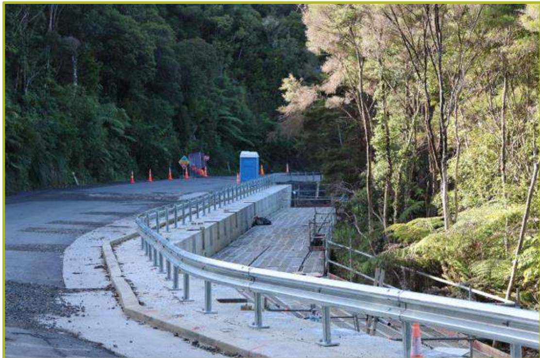
Figure 7: Example of Typical Slip Site (Slip A3 Near Completion of Remediation Works (Image Taken: 14 August 2024))
