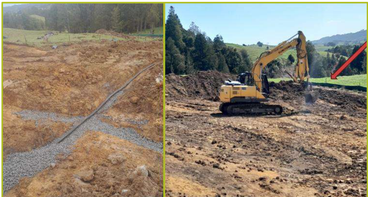
Figure 19: (Left) Subsoil Drainage being Installed; (Right) Silt Fence around the perimeter
