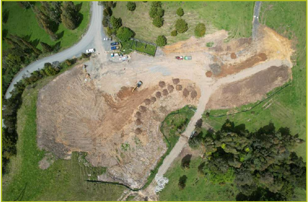
Figure 2: Aerial Image of Site near completion of works (Image taken 29 October 2024)
