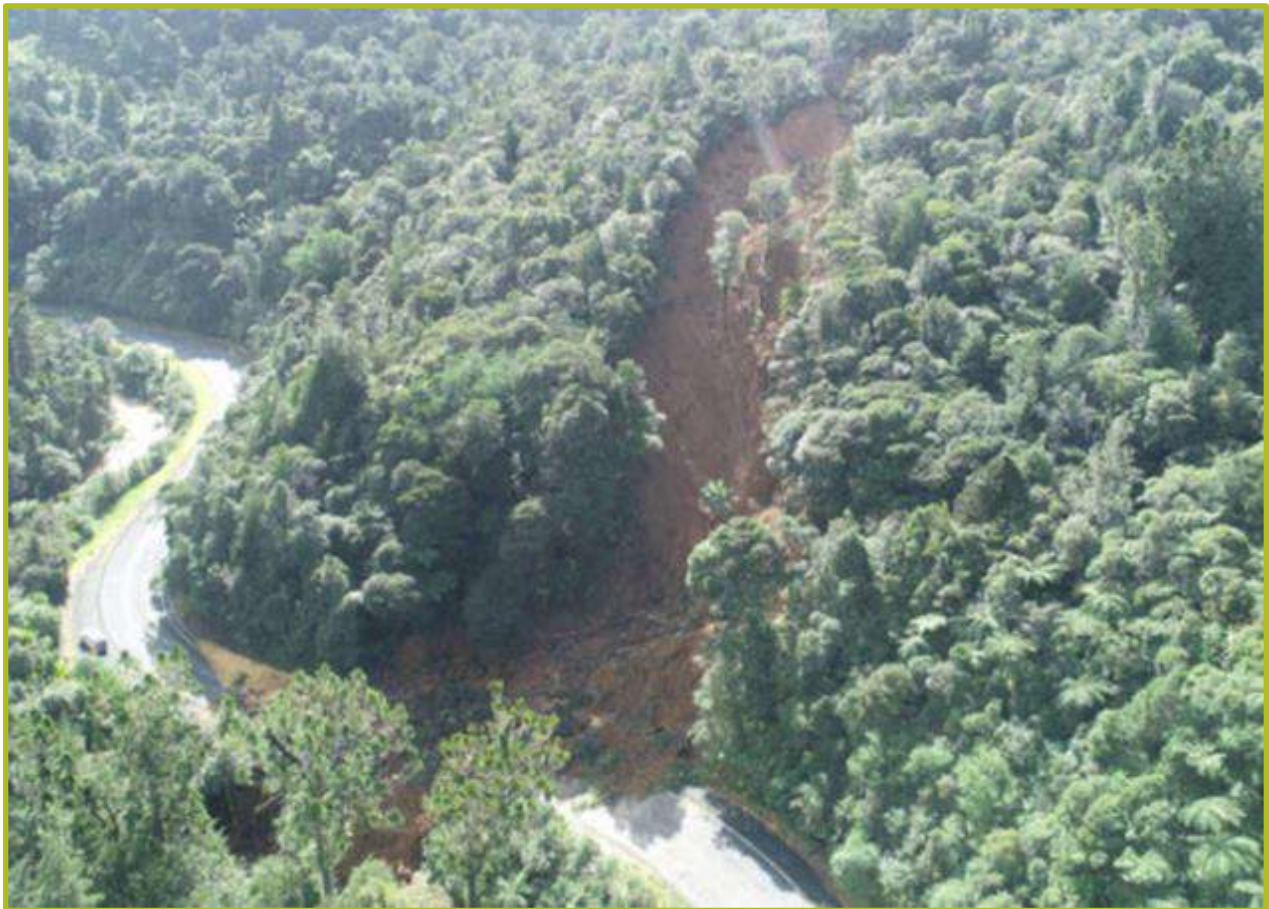
Figure 2: A large slip at the southern end of the Gorge in the immediate aftermath of 19 August 2022 Weather Event (Source: NZTA Media Release - 24 August 2022)
