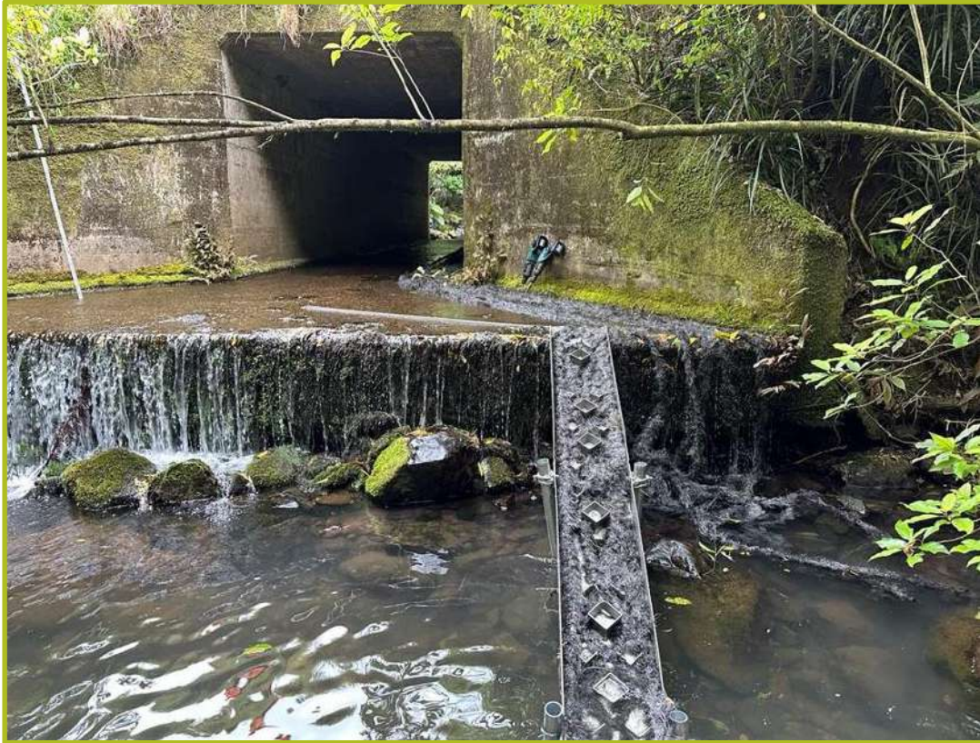
Figure 9: Fish Ladder installed as part of the Fish Passage Betterment across the Gorge (Image taken 5 December 2024)
