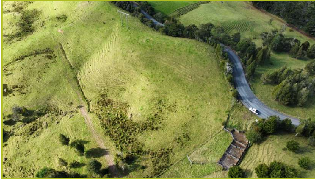
Figure 4: Aerial Photo showing location of cleanfill site taken prior to works being undertaken
