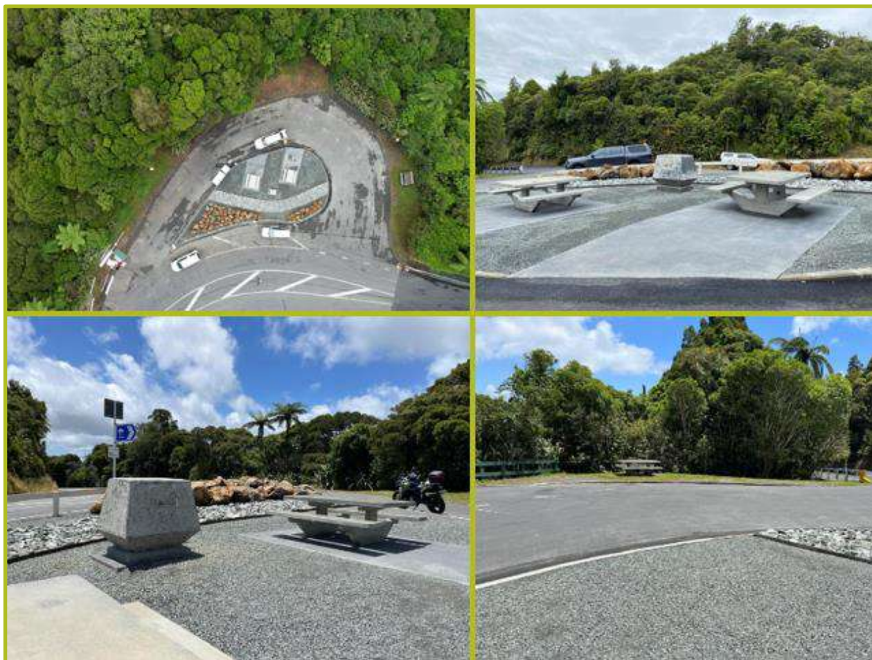
Figure 11: "Rest Area" constructed at the Mangamuka Gorge Summit
