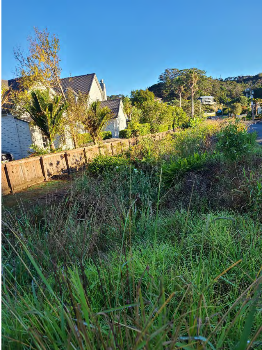
Figure 2 Main stormwater drain in Beresford St
