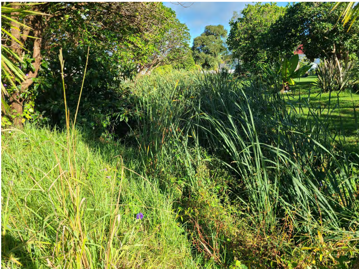
Figure 1 Main stormwater drain through town by Medical Centre
