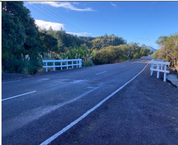
7-23-102 Whangaroa, Waharua & West Coast Road Culvert Renewals - Whangaroa
