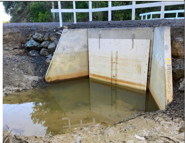
7-23-102 Whangaroa, Waharua & West Coast Road Culvert Renewals - Whangaroa
