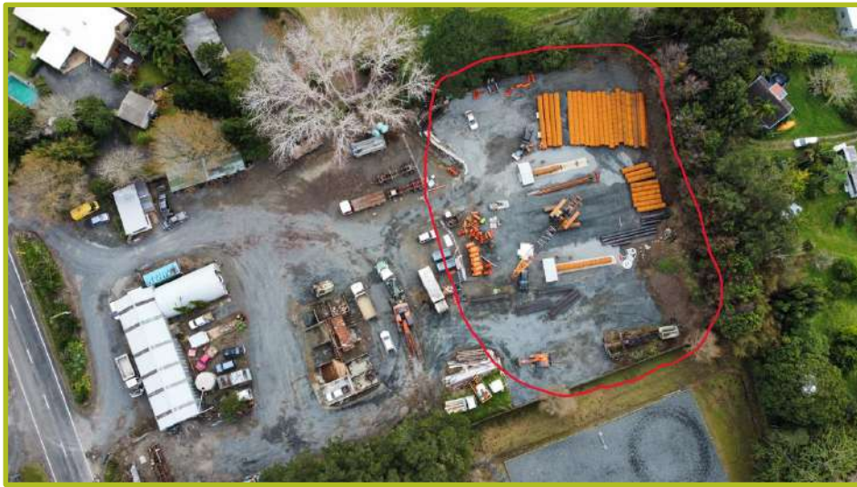
Figure 8: Northern Laydown Area (red square) Drone Photo
