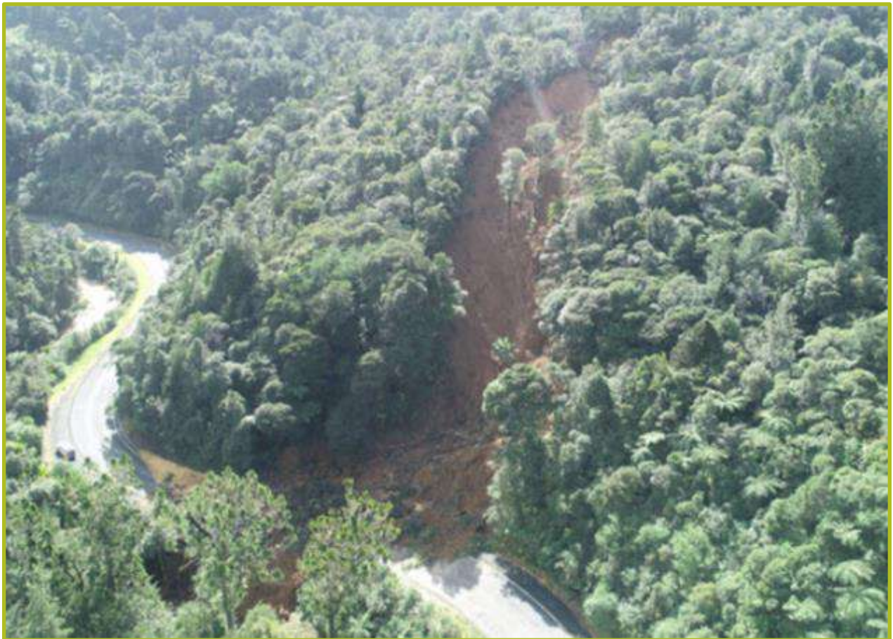
Figure 2: A large slip at the southern end of the Gorge in the immediate aftermath of 19 August 2022 Weather Event (Source: NZTA Media Release - 24 August 2022)
