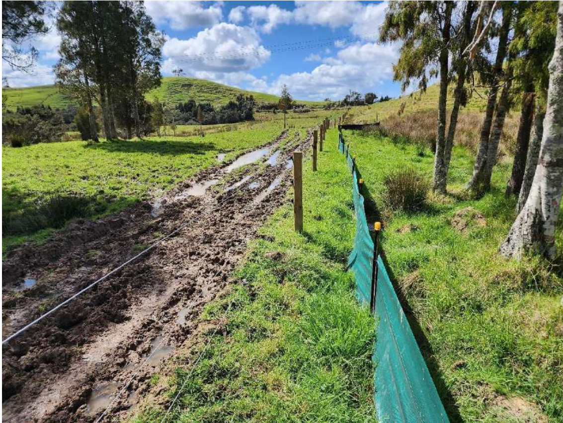
Figure 75: Looking northeast along farm track/old road alignment.
