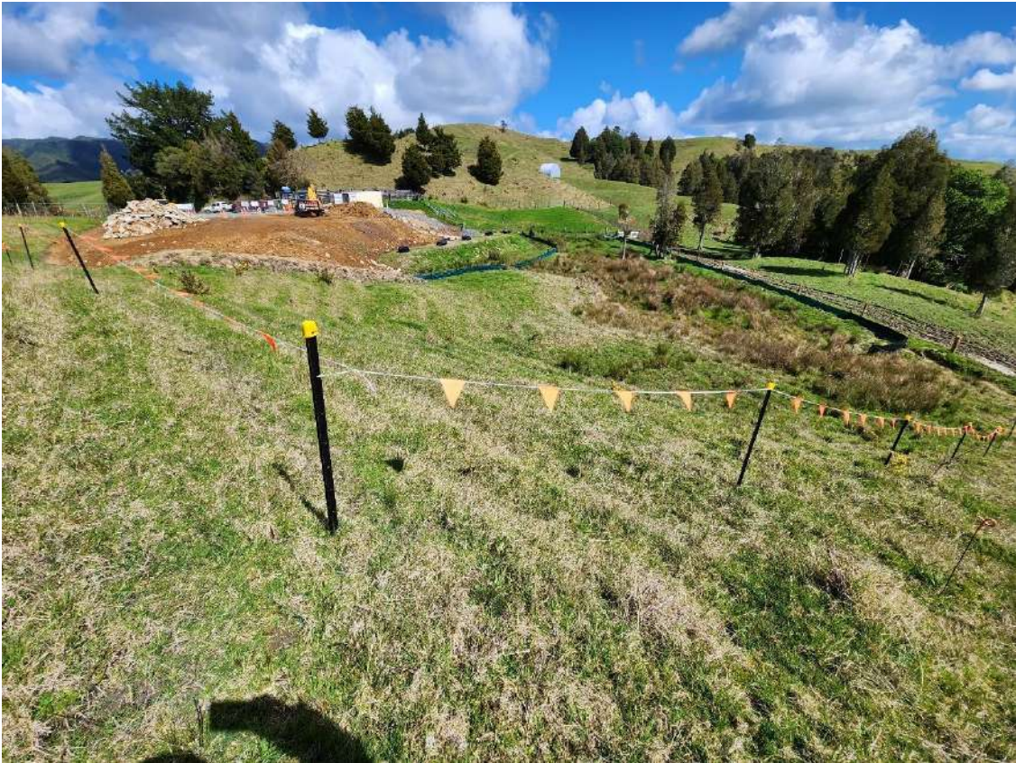
Figure 73: Peria Valley Road spoil dump site, looking west.
