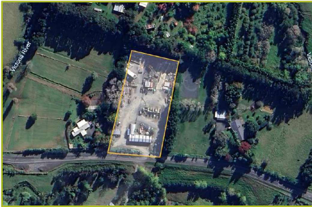
Figure 2: Aerial Image of 6770 State Highway 1 (Source: GoogleEarth - accessed 25 November 2024)
