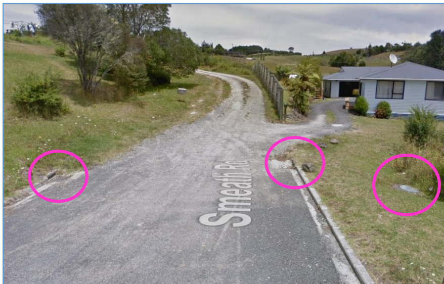
Figure 12: Existing SW Asset Locations on Smeath Road shown Google Street View
