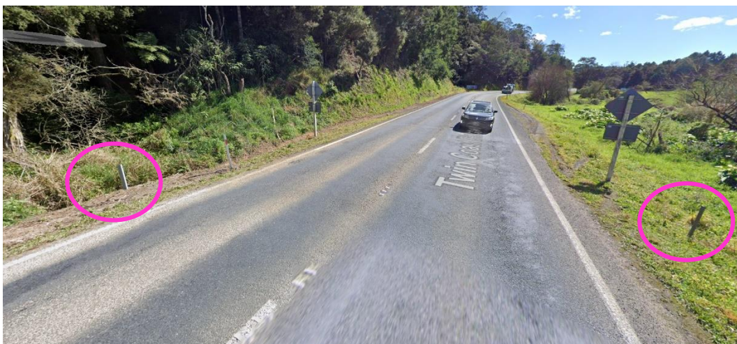
Figure 8 Culvert under State Highway 1 shown on Google Street View
