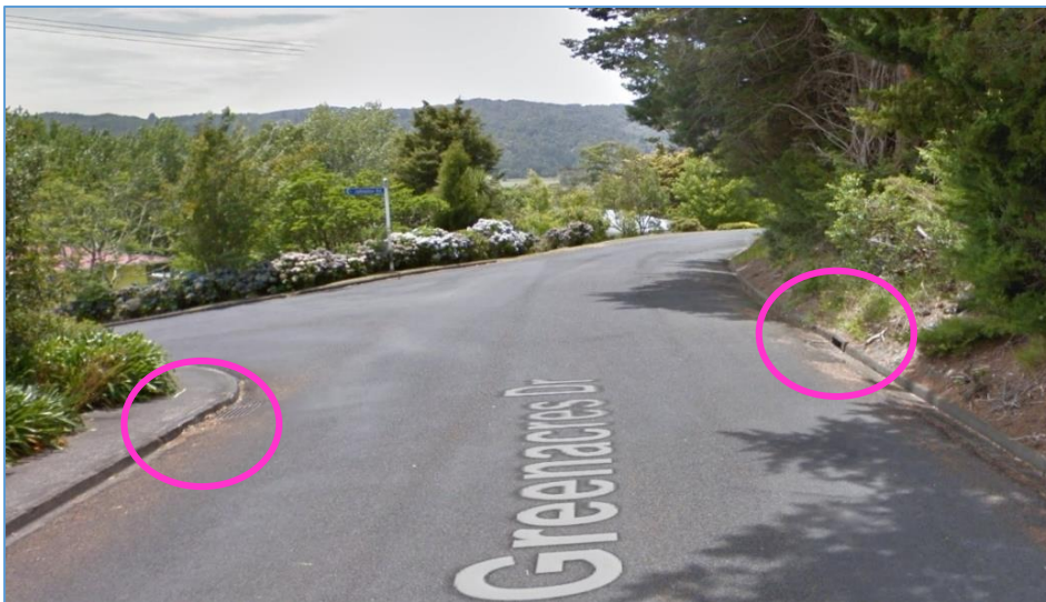
Figure 6: Existing Catchpit Locations on Greenacres Drive shown on Google Street View
