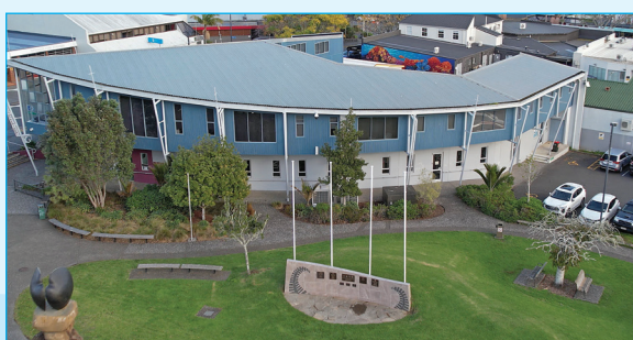
Renovations will boost council services at Procter Library.
