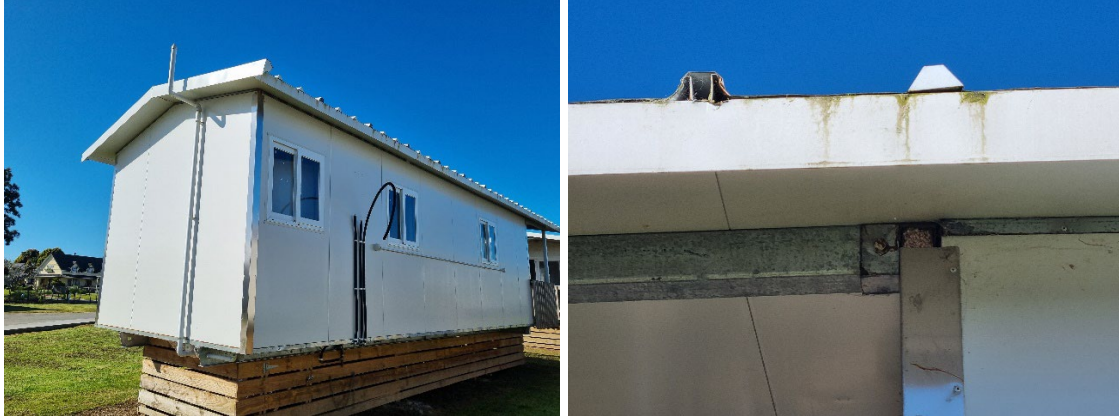
Figure 7: Roof cladding and soffit linings
