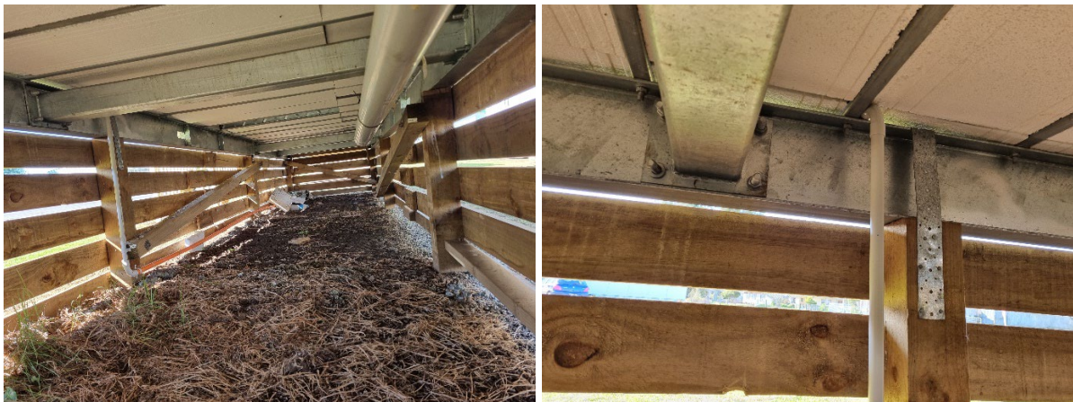
Figure 4: Subfloor framing
