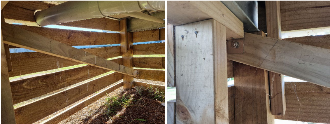
Figure 5: Subfloor bracing
