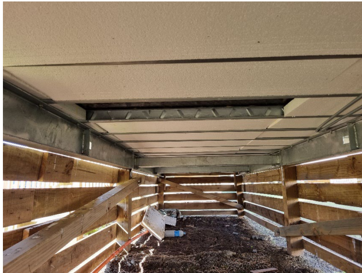
Figure 13: Underfloor insulation
