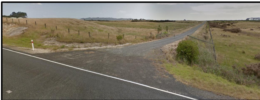
Figure 8: Image of existing crossing place and private accessway from Inland Road.
