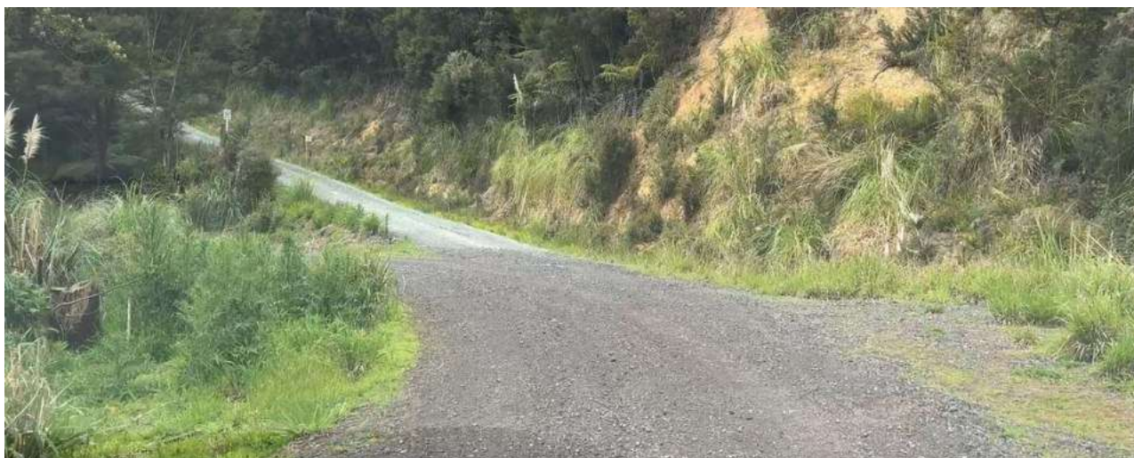
Photo 9. Looking east along Te Raupo Road from 1680 metres; another existing passing bay and the start of the shared access (on the rise). Stabilisation of the access pavement is proposed where the gradient is steeper than 20%, which occurs in some of this section (on both sides of this hill and on for a short distance east of the cycle trail (see photo 16).
