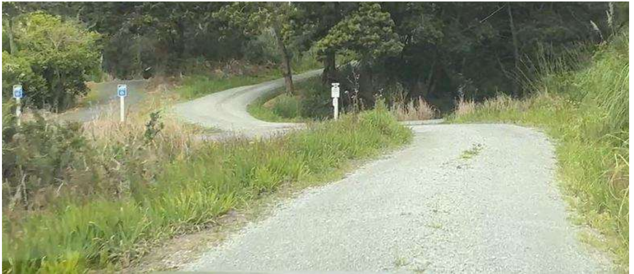
Photo 14. Looking northwest along the shared access and across the cycle trail/rail crossing. The original trail runs from left to right, but the section at left, which leads to tunnel, has been bypassed by a temporary trail, part of which is visible at right. As such, until the tunnel is re-opened, there is no conflict with cyclists at this crossing.
