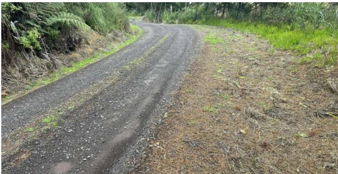
Photo 3. Another existing passing bay on Te Raupo Road.
