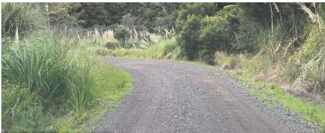
Photo 9. Looking east along Te Raupo Road from 1680 metres; another existing passing bay and the start of the shared access (on the rise). Stabilisation of the access pavement is proposed where the gradient is steeper than 20%, which occurs in some of this section (on both sides of this hill and on for a short distance east of the cycle trail (see photo 16).
