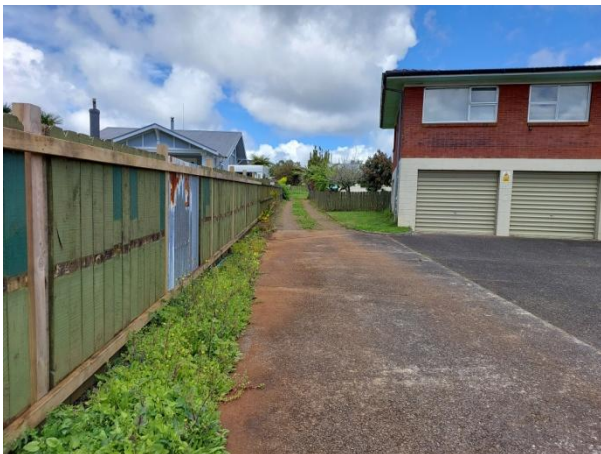
House in the foreground is the dominant tenement for the ROW.
