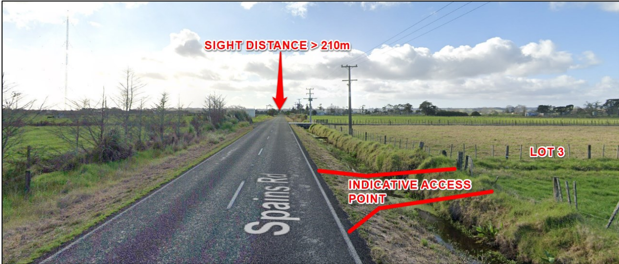
Figure 11: Indicative Access Point on Spains Road Facing East, >210m Sight Distance Available.
