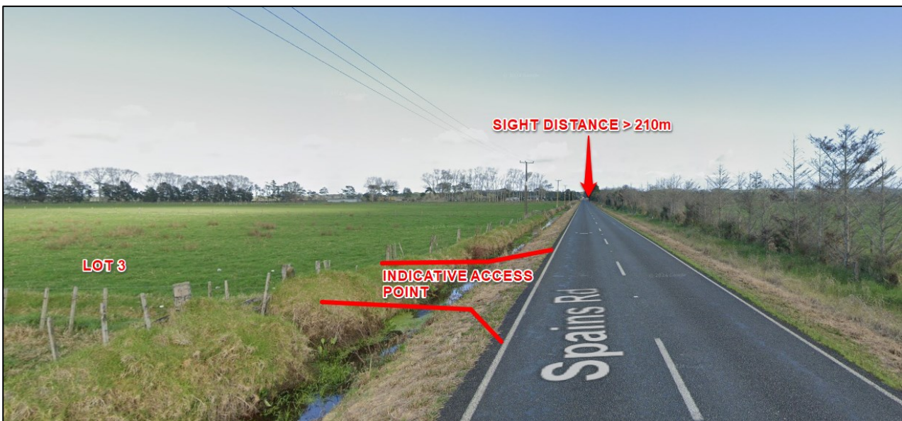
Figure 12: Indicative Access Point on Spains Road Facing West, >210m Sight Distance Available.
