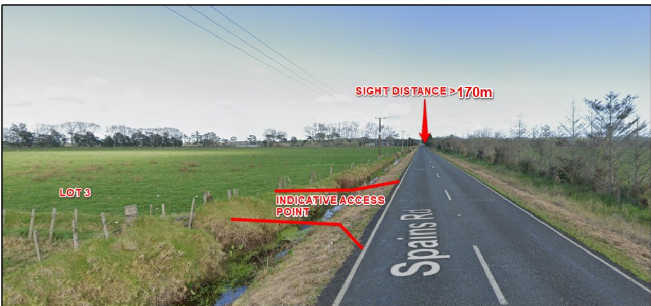
Figure 12: Indicative Access Point on Spains Road Facing West, >170m Sight Distance Available.
