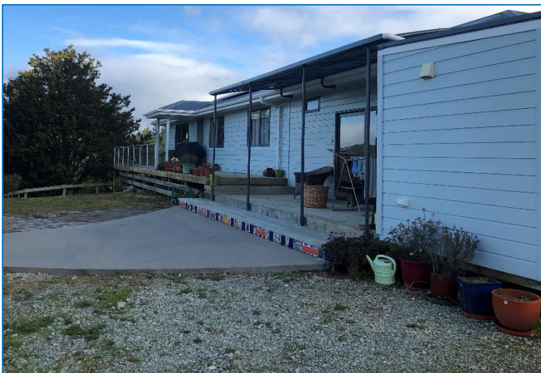
Photograph 1: Existing building – Lot 1.
